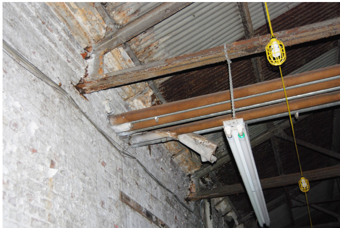
Existing Conditions Photos: Trusses at Shed Hitting Protected Structure
