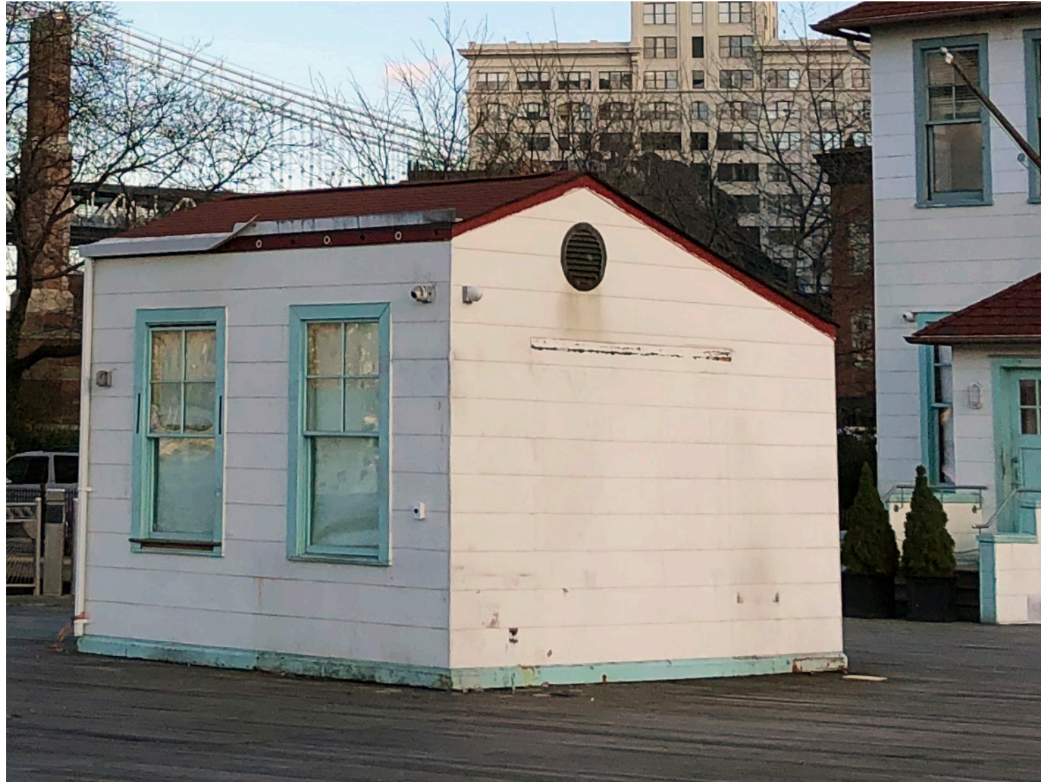
Current Condition of Hose Shed | South and West Facades January 2019
