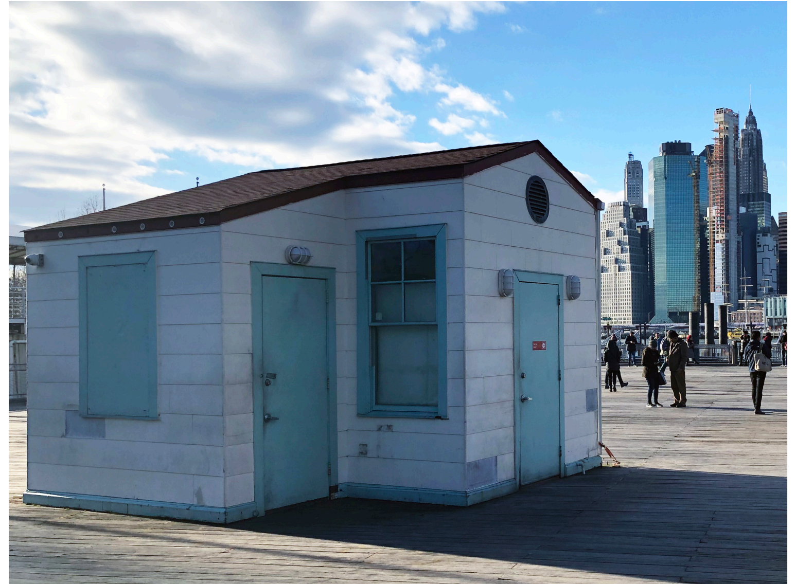
Current Condition of Hose Shed | North and East Facades January 2019
