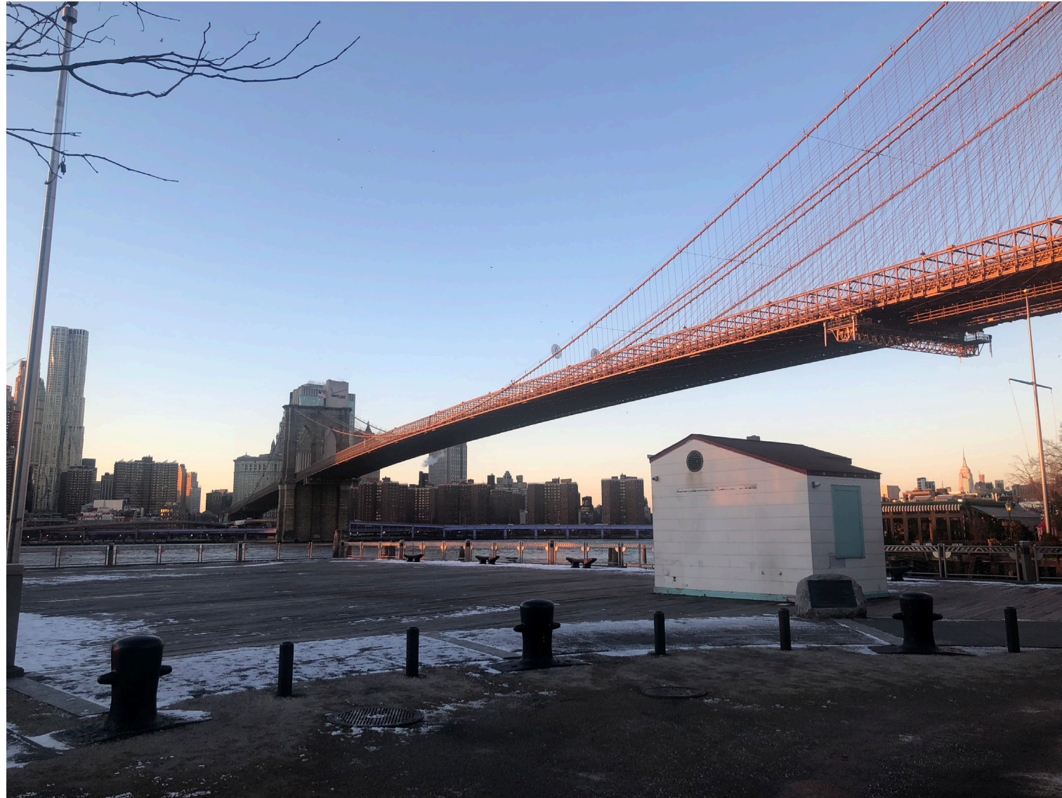
Current Condition | View looking towards the Brooklyn Bridge January 2019
