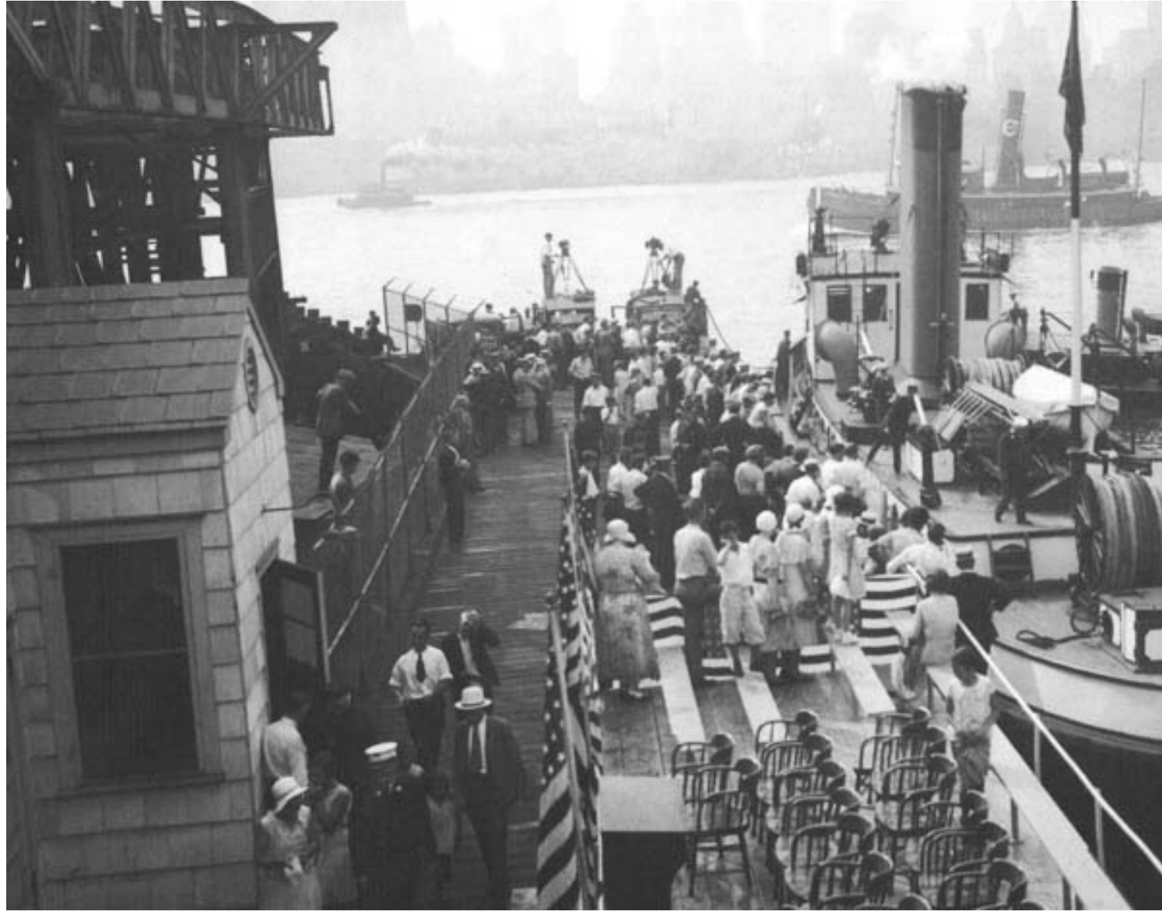
Hose Shed with Shingles and Slate Roof July 28, 1931
