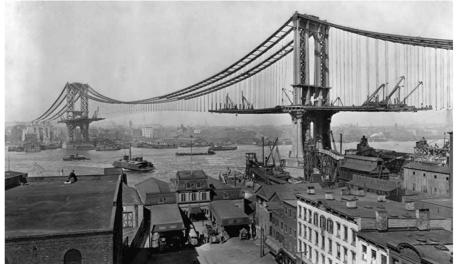
View of the Manhattan Bridge Under Construction 1909
