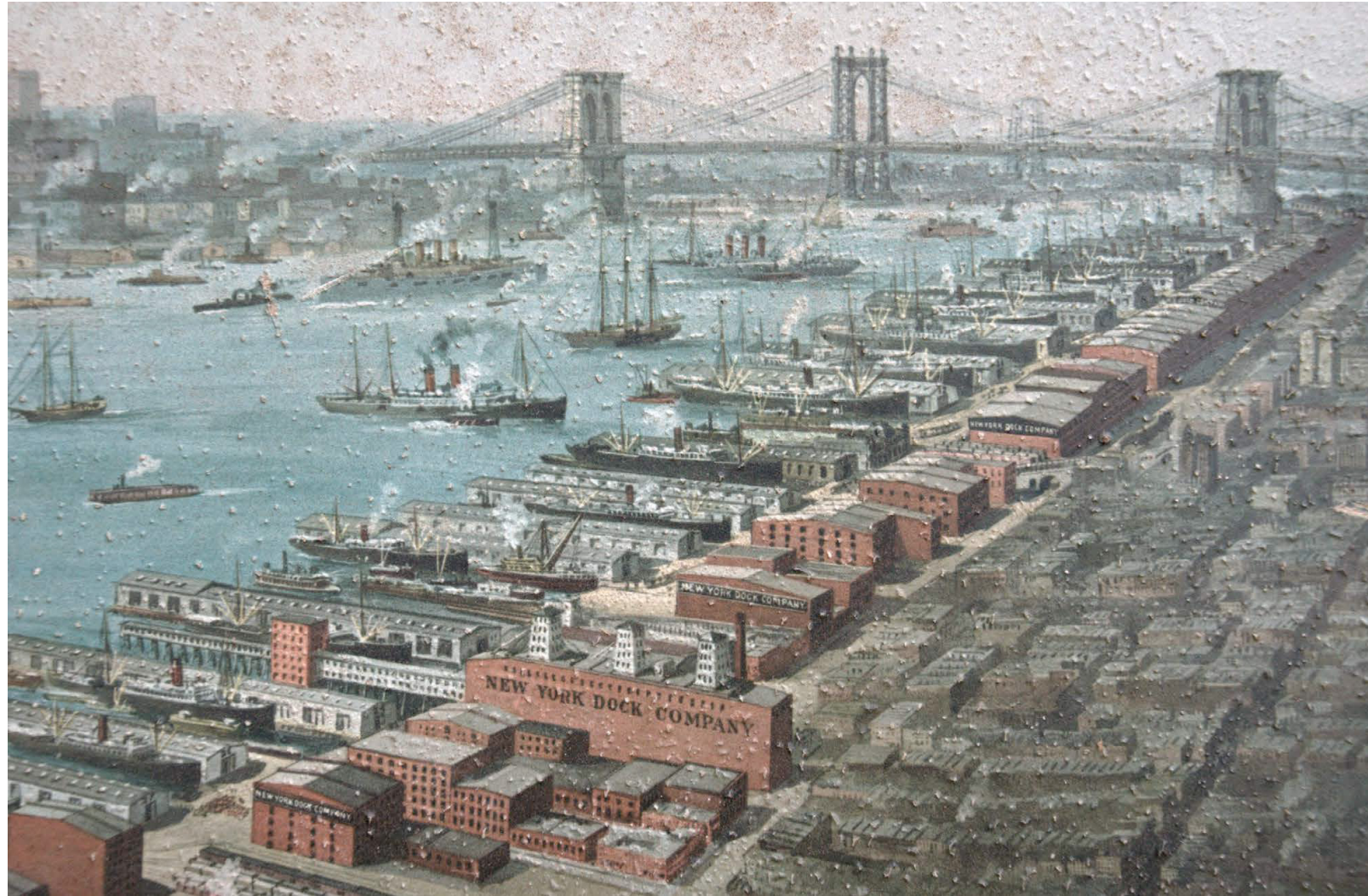
Illustration of the Brooklyn Bridge and Fulton Ferry Landing ca. 1911
