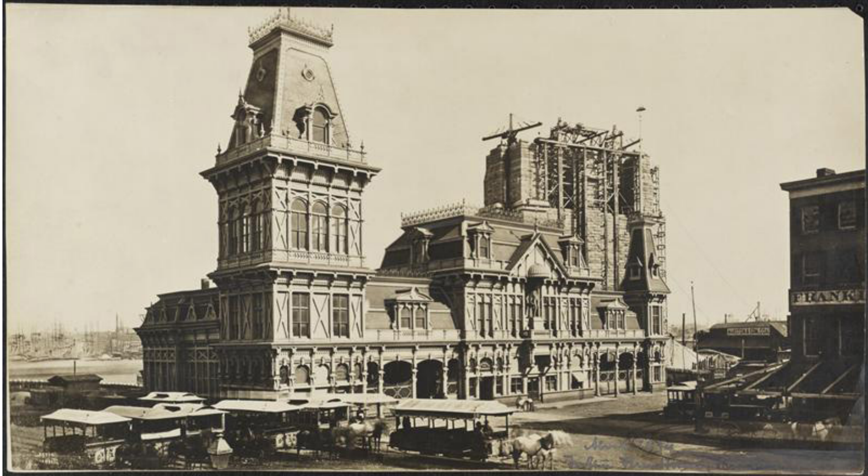
Fulton Ferry Terminal with the Brooklyn Bridge under construction Peter Juley
