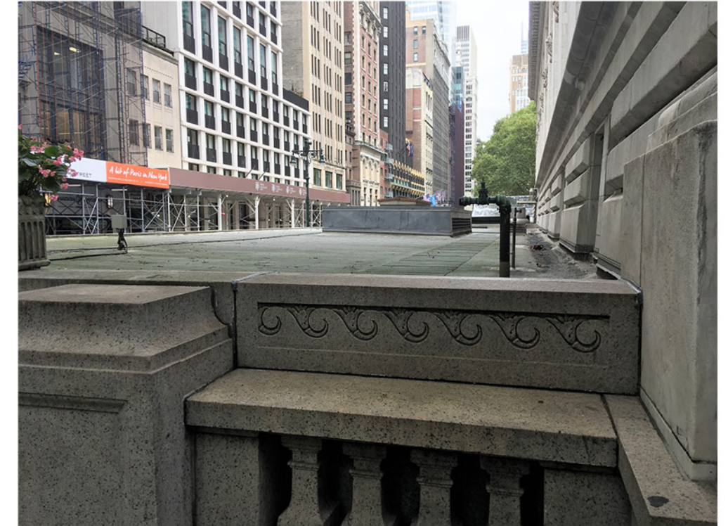
▲ 3 Existing roof over electrical room
