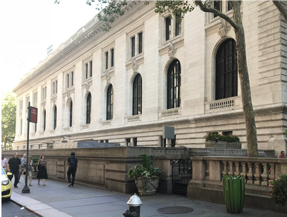
▲ 1 Existing street wall at 40th Street
