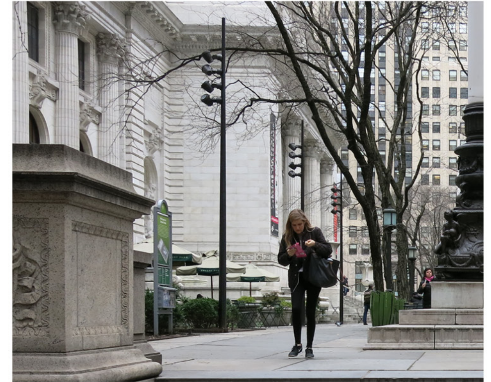
▲ Pole lighting, installed c. 2010
