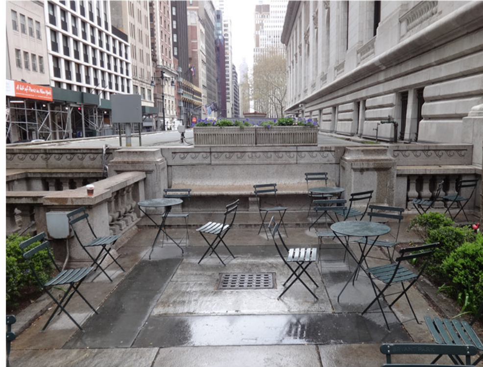
▲ 2 Existing bench & engaged piers
