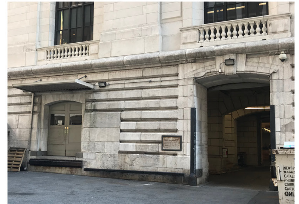
▲ Existing surface-mounted lighting at Loading Dock
