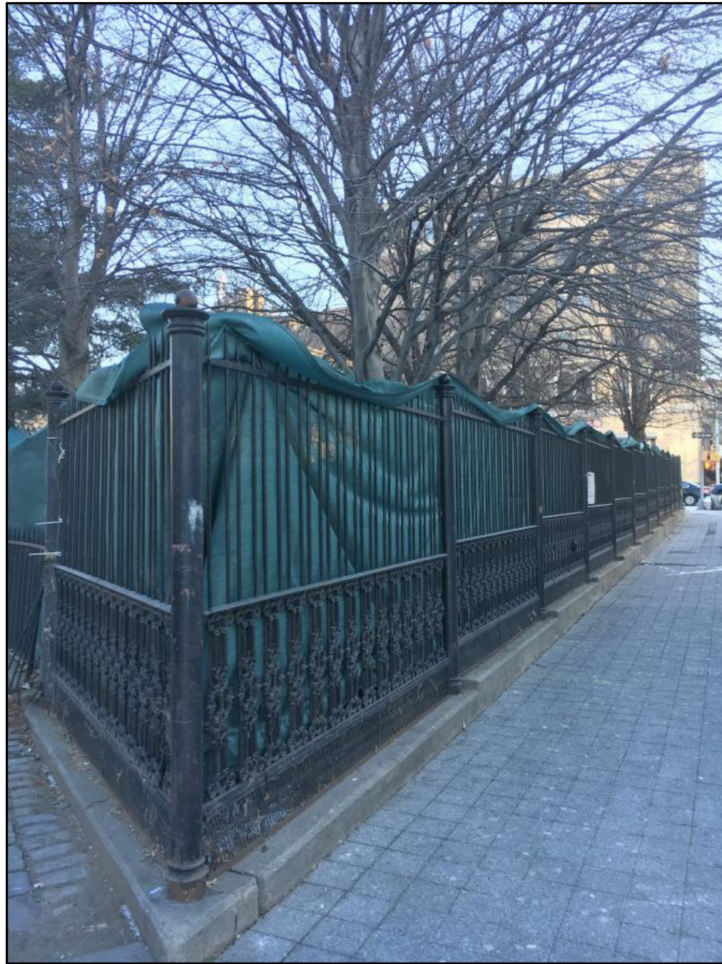
VIEWING SOUTH FROM CORNER OF FULTON ST AND ST FELIX STREET
