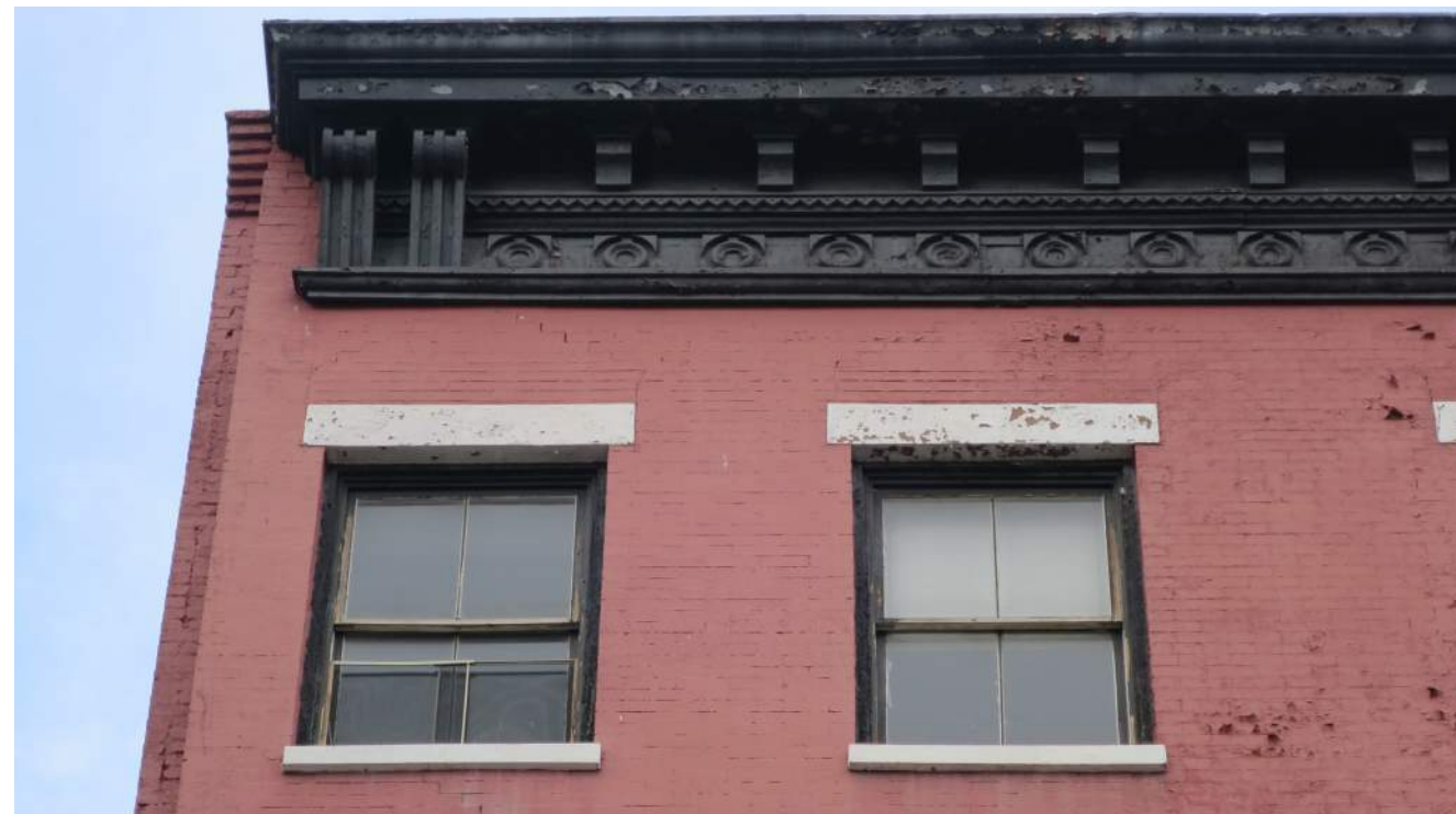
HISTORIC METAL CORNICE AND DETERIORATED WOOD WINDOWS
