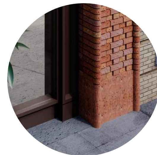
DETAIL 1: PIER BASE & STOREFRONT COLUMN
