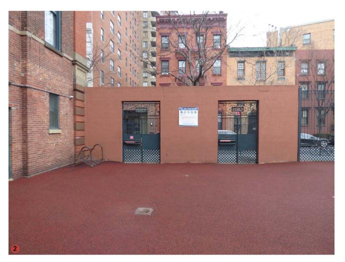
Rear view of the wall, constructed of CMU, with brick and cast stone outer face.
