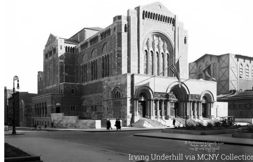
North West Corner ca. 1919
