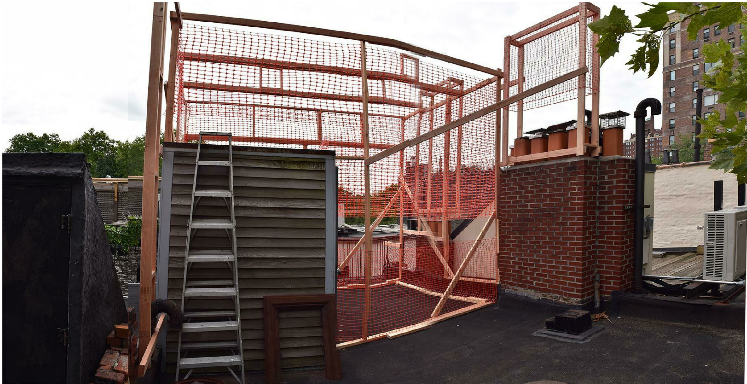
MOCK-UP PICTURE VIEW FROM THE ROOF
