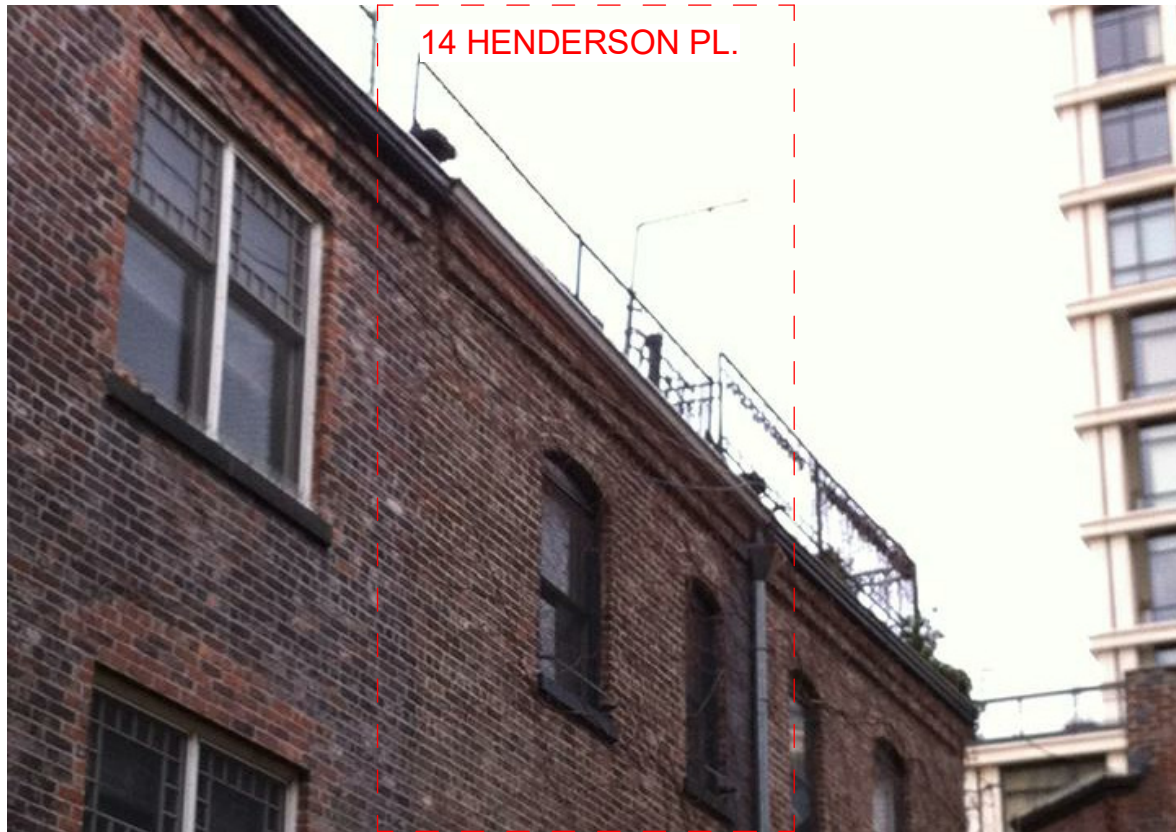
EXISTING BACK FACADE CORNICE AND GUTTER
