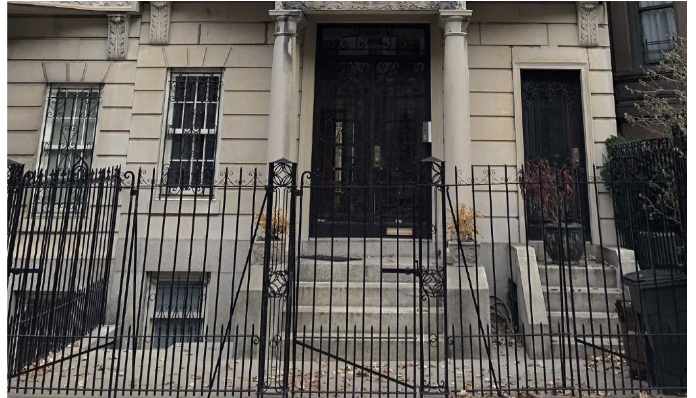
ENTRY AREAWAY - BEFORE
