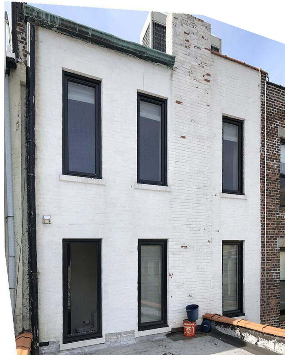
Existing Upper Rear Facade Photo
