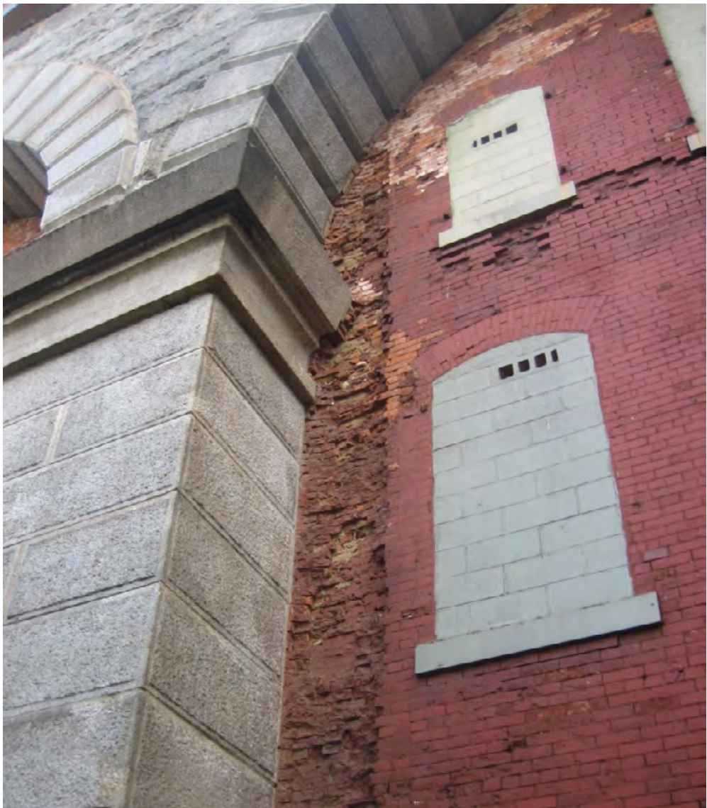
2- Deteriorated Brickwork on Exterior Arch Infill Wall
