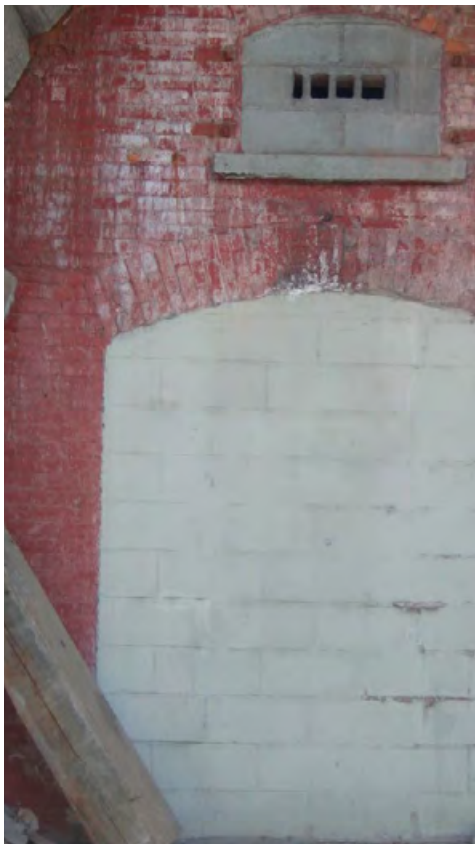
6 - Brick Round Arch with Straight Brick Voussoirs IMG_5949
