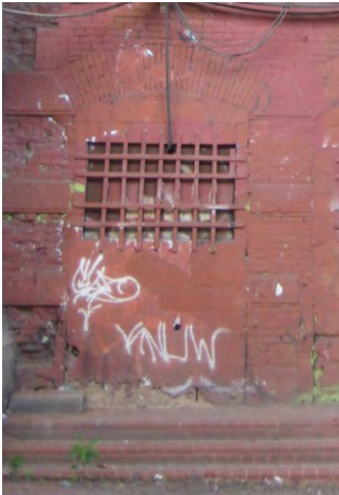
2 - Infilled Opening with Metal Security Grate
