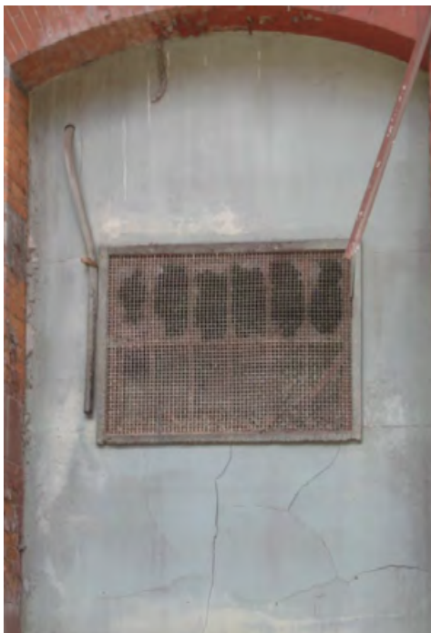
4 - Metal Window with CMU Infill
