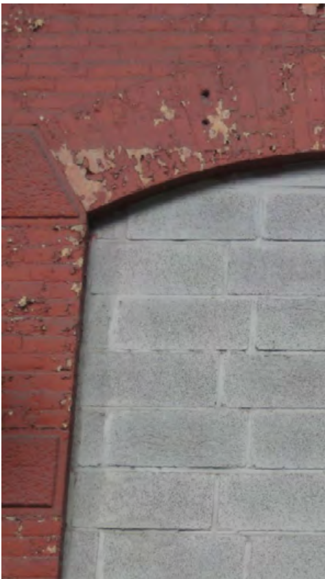
4 - Brick Segmented Arches with Bullseye Brick Voussoirs IMG_5889
