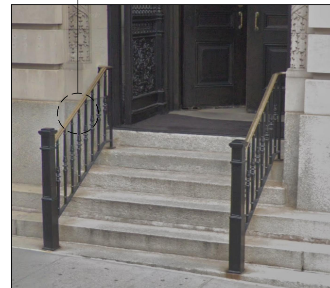
240 CENTRE STREET - RAILING
