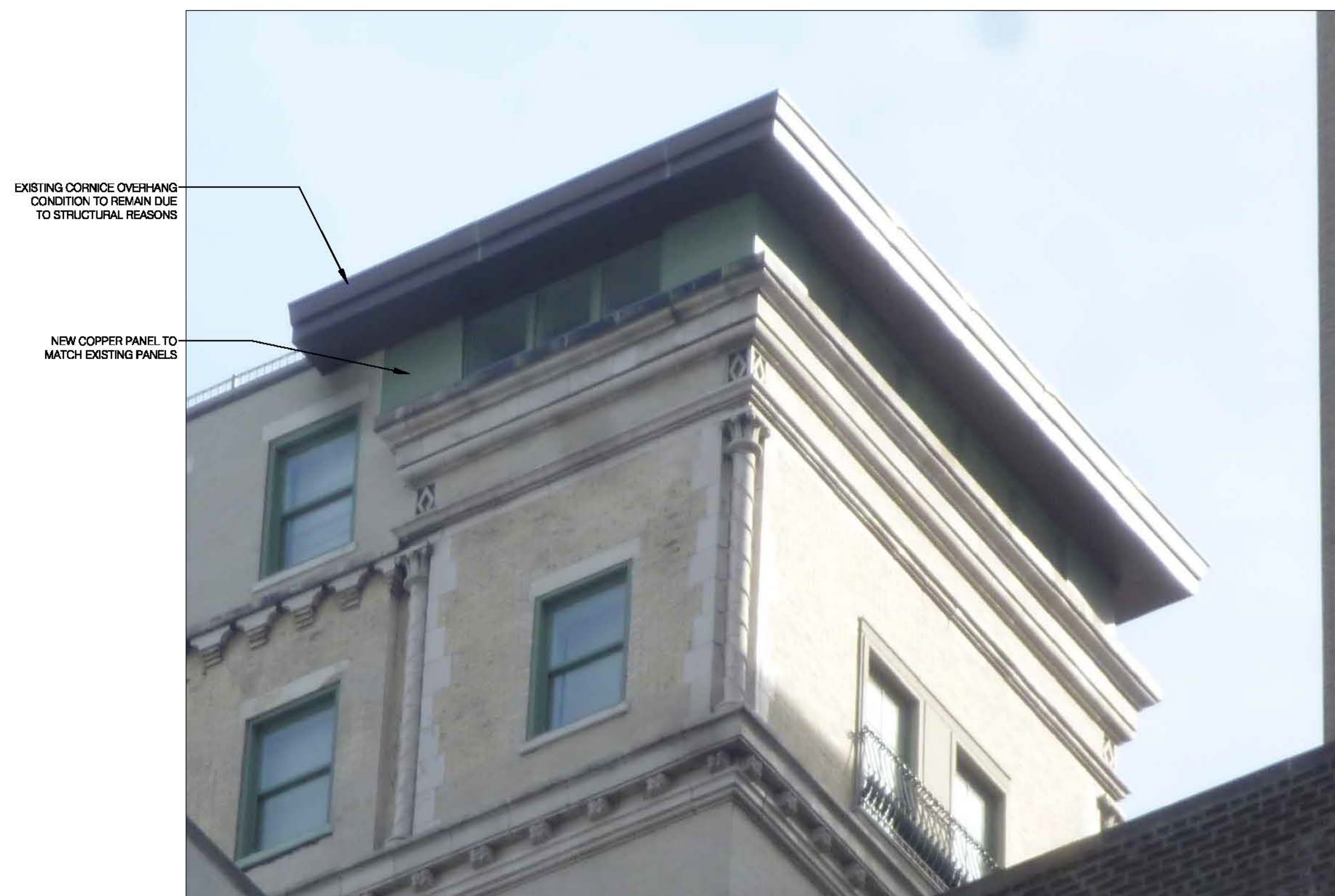
3 PROPOSED NW TURRET BUILT CONDITION A-501 SCALE: NTS
