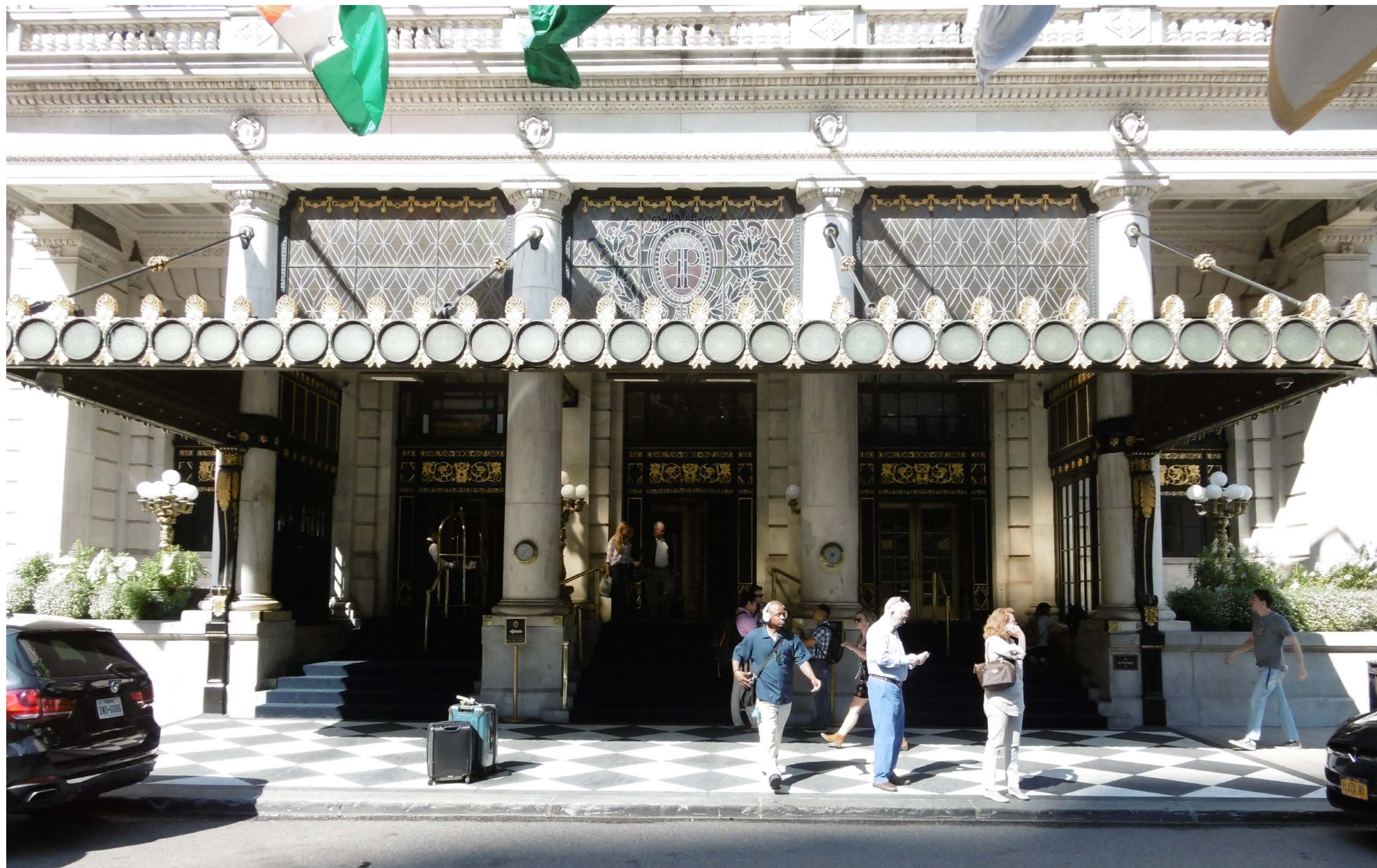
5TH AVENUE AWNING
