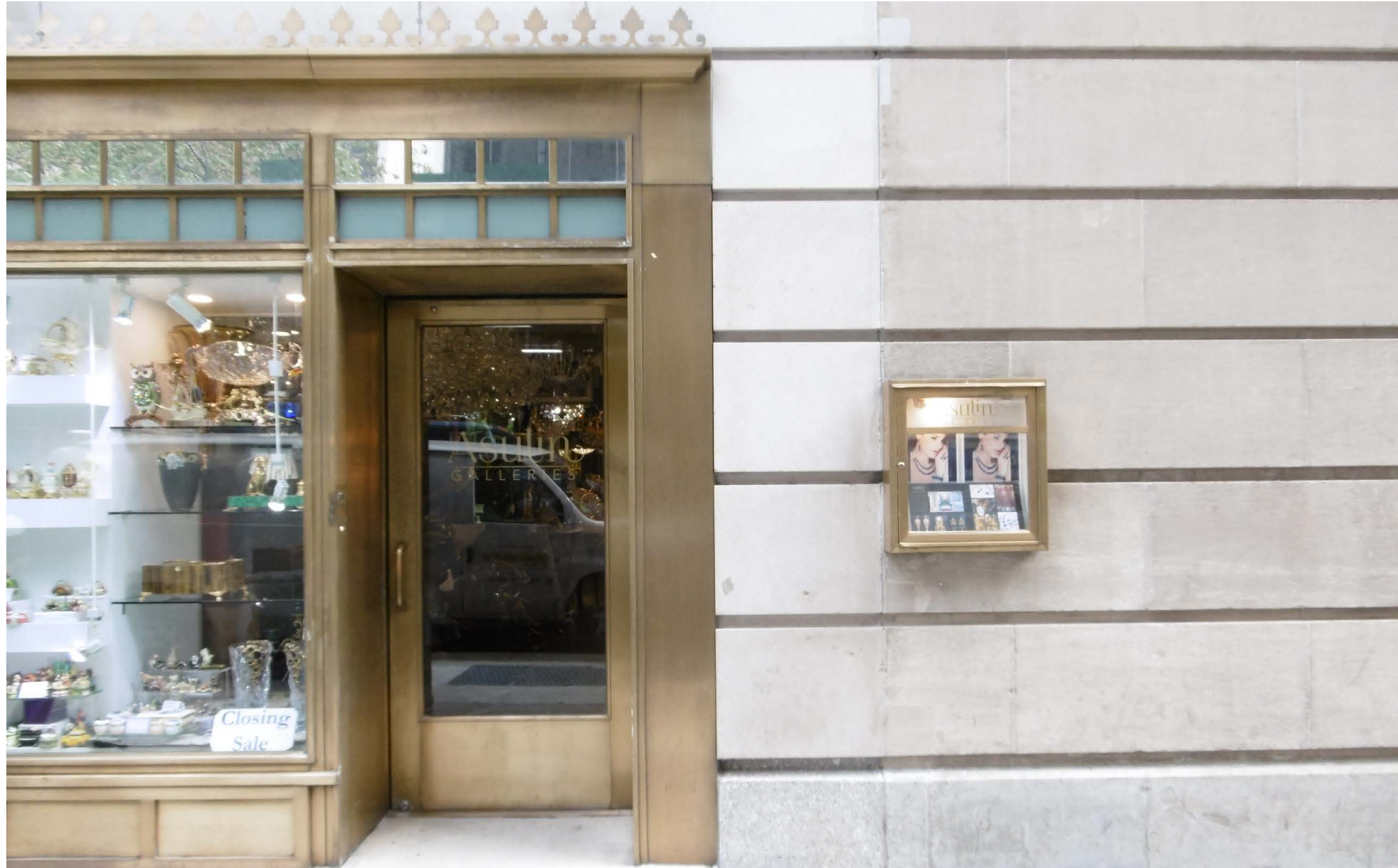
58TH STREET STOREFRONT ENTRY
