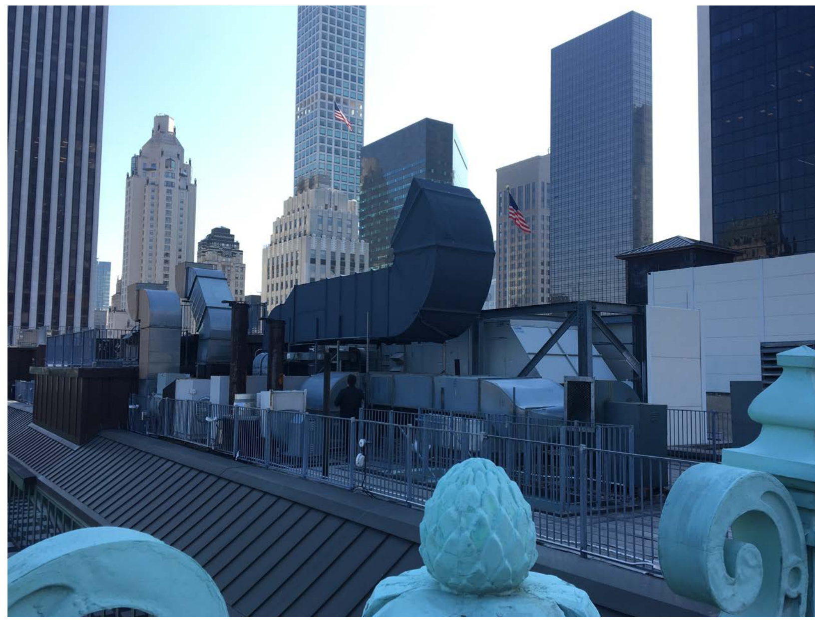
1. VIEW FROM NW CORNER FACING SE
