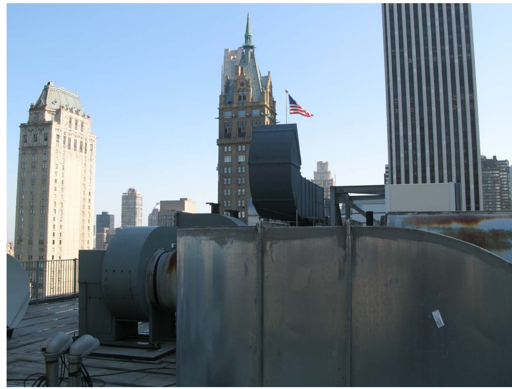
2. VIEW FROM WEST FACING NE
