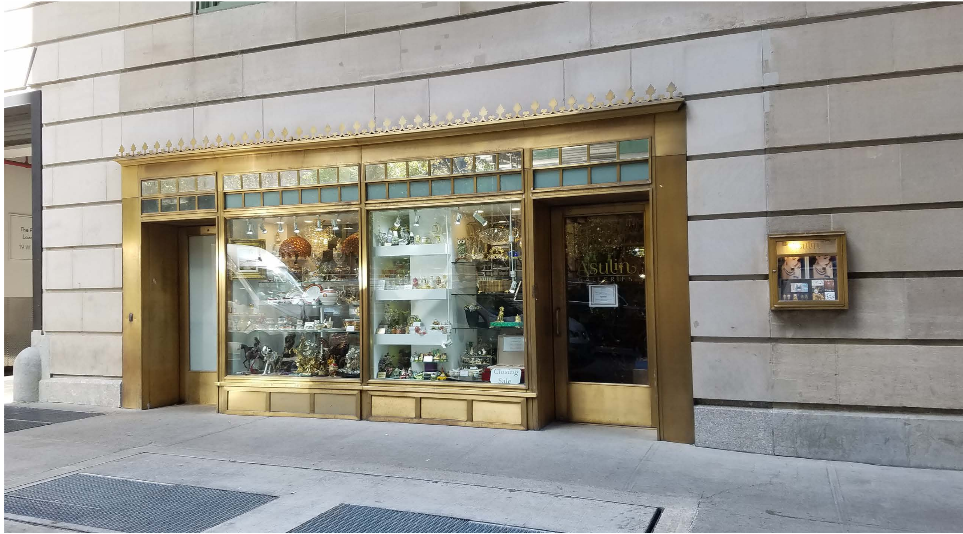
58TH STREET STOREFRONT
