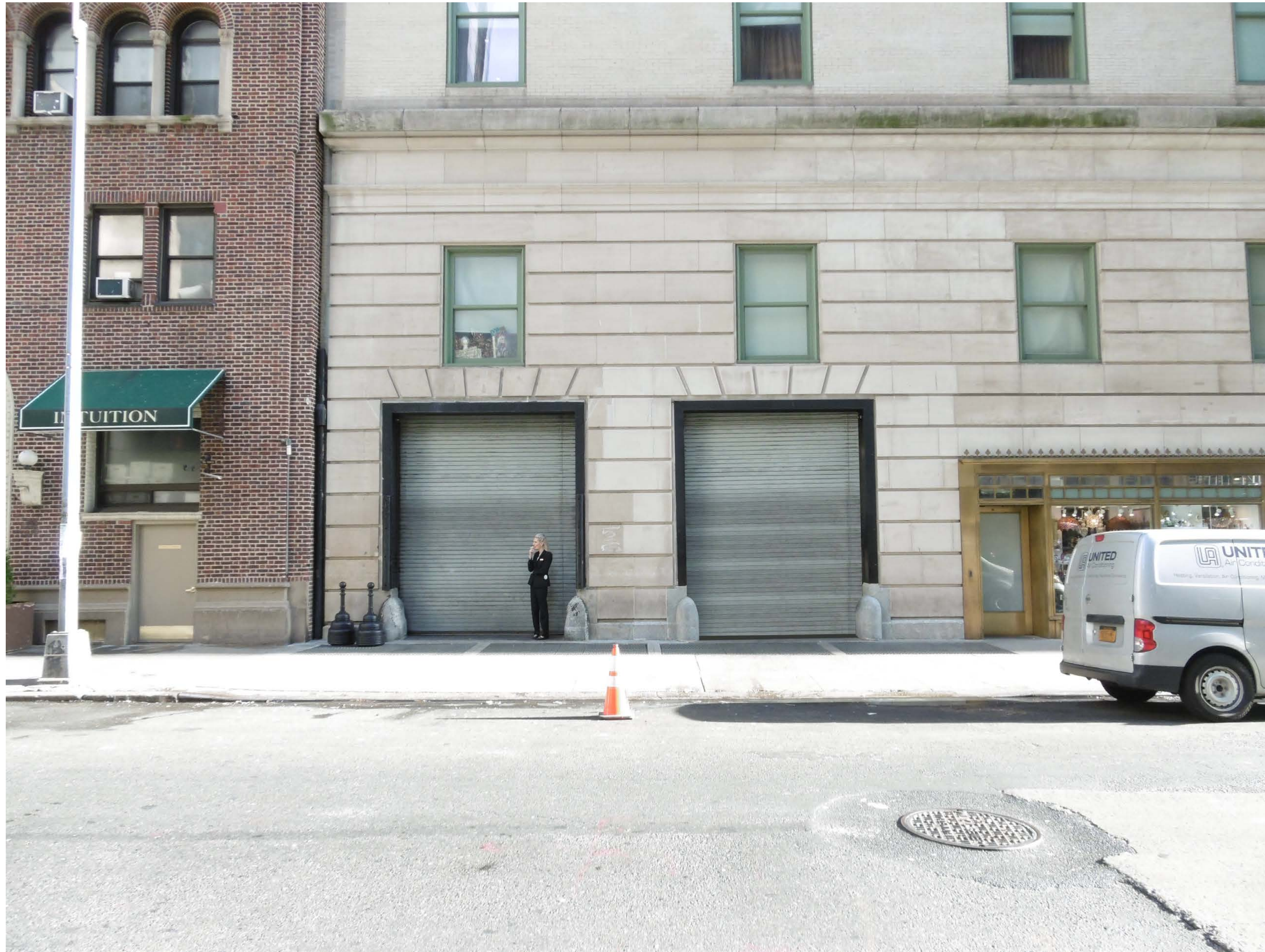
EXISTING LOADING DOCK DOOR PHOTO
