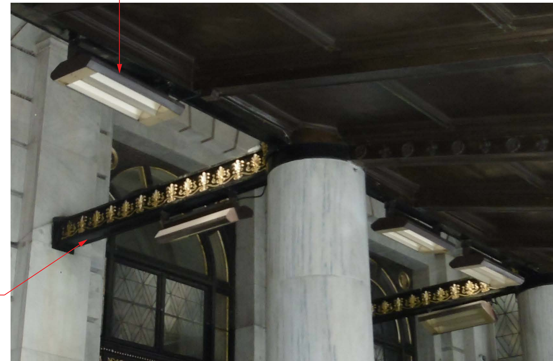
EXISTING PHOTO OF 5TH AVENUE AWNING
