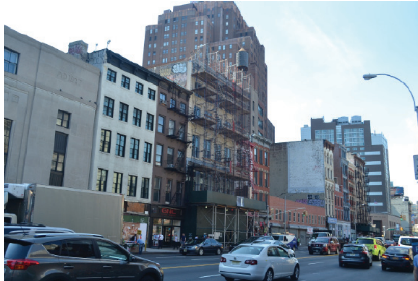
From East on Canal
