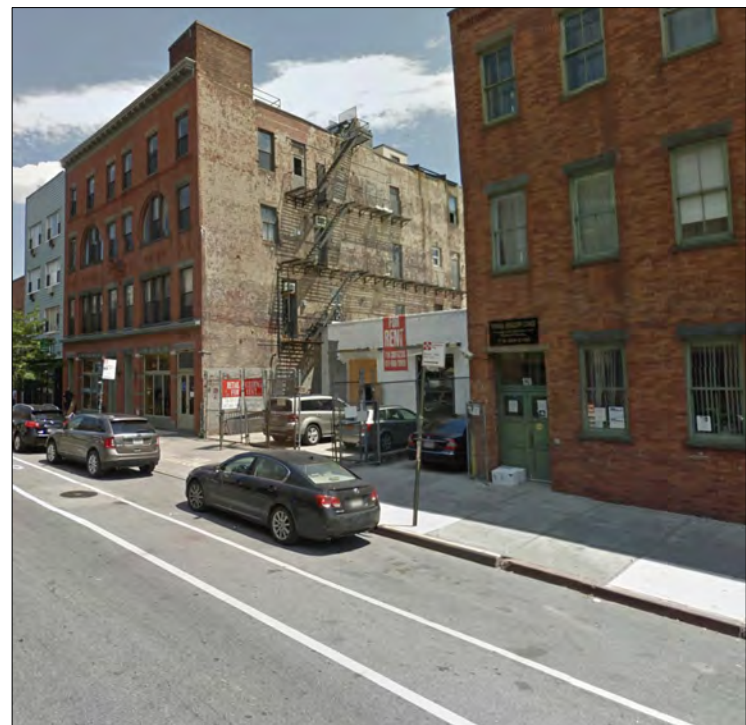
EXISTING VIEW LOOKING WEST
