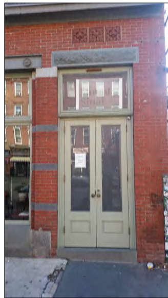
132 GREENPOINT AVENUE EXISTING FACADE
