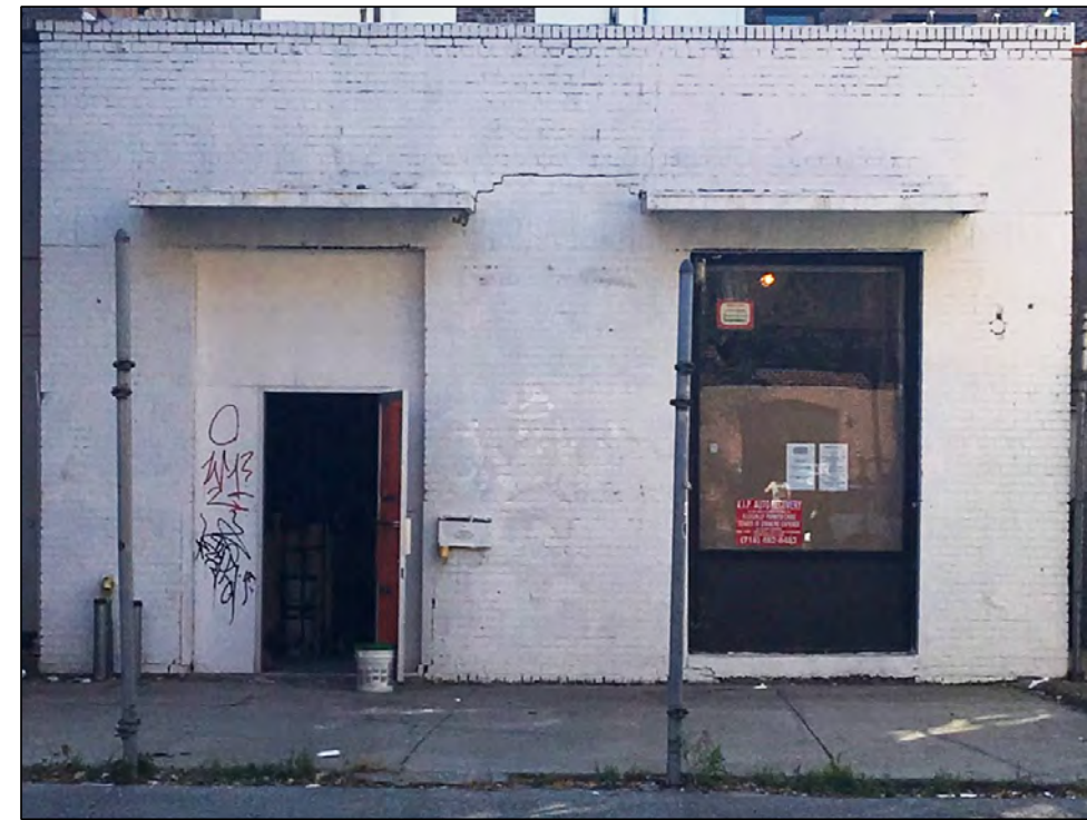
DETAIL VIEW OF EXISTING FACADE
