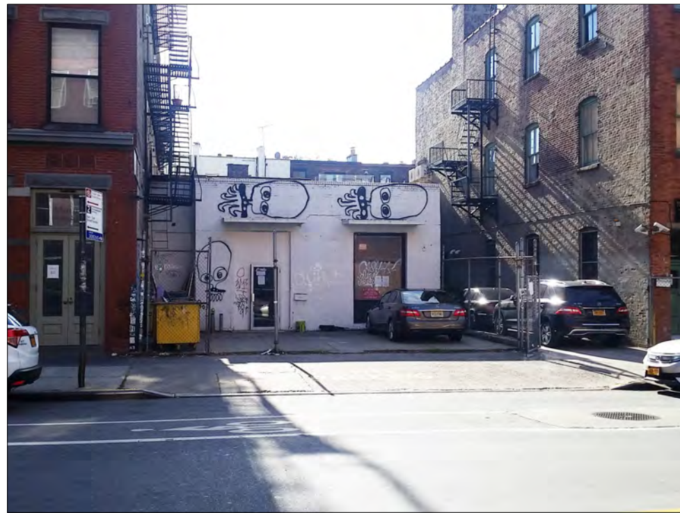
EXISTING FACADE VIEW FROM ACROSS GREENPOINT AVE
