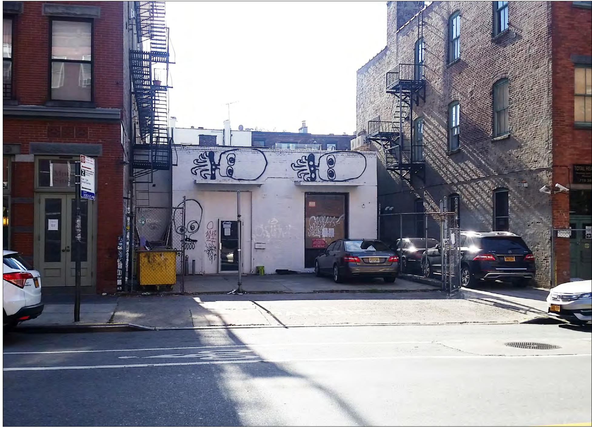
EXISTING VIEW FROM GREENPOINT AVENUE
