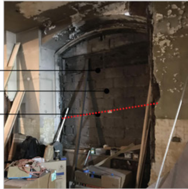
EXISTING CONDITIONS AT WINDOW 8 SIMILAR FOR WINDOWS 6,7,9
