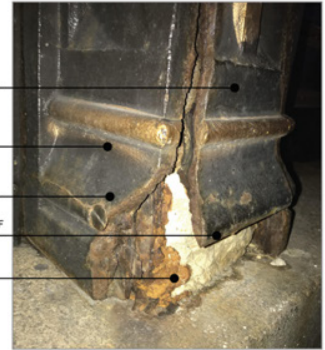
EXISTING CONDITIONS AT WINDOW 12
