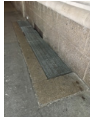
3. EXISTING RECESSED WINDOW WELL
