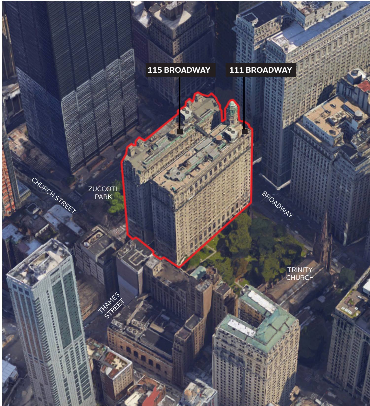
111 - 115 BROADWAY SOUTH WEST AERIAL VIEW
