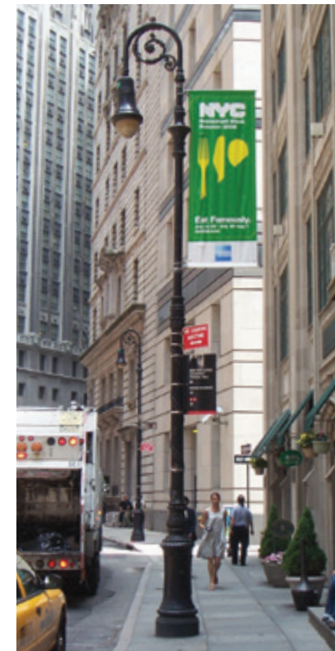
Historic Bishops Crook luminaire and pole: Nassau Street, Manhattan
