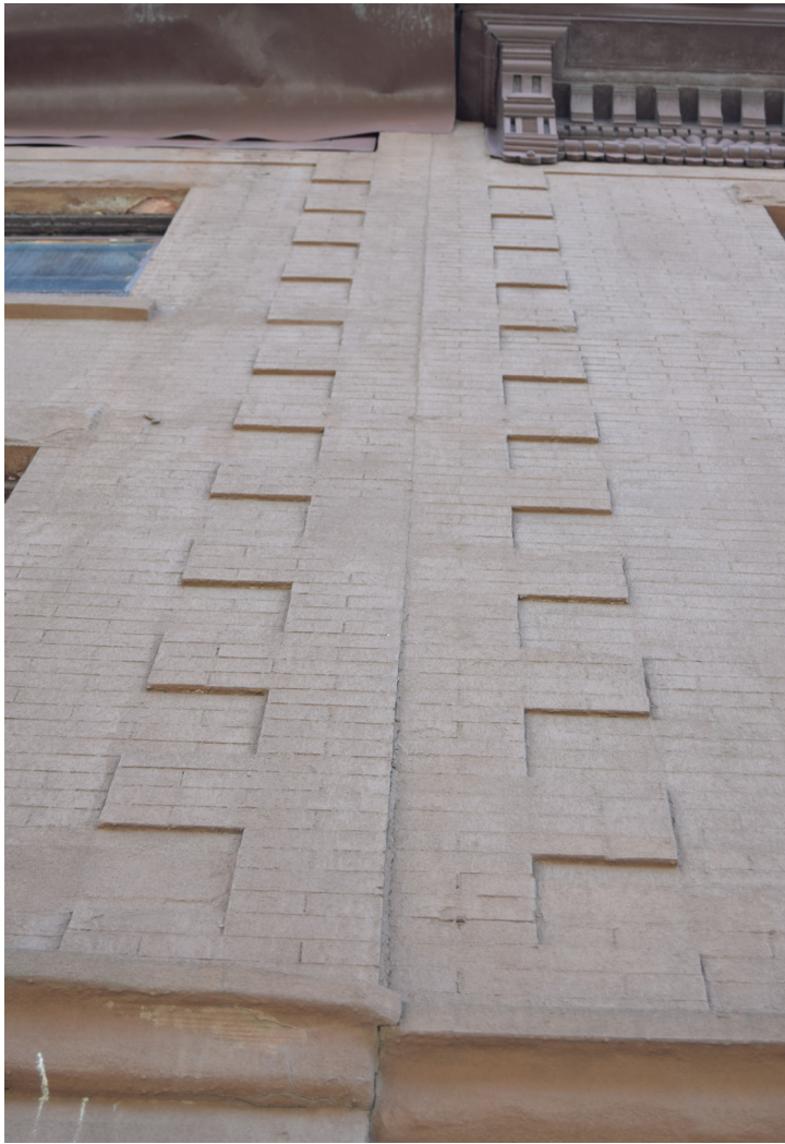
A. BRICKWORK QUOINING DETAIL
