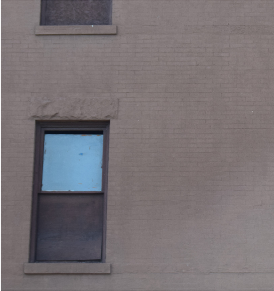
A. BRICK FAÇADE WITH STUCCO TOP COAT
