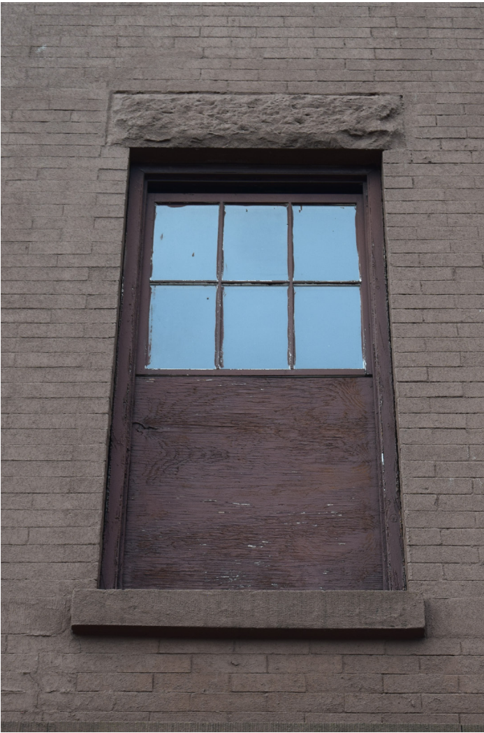
B. WINDOW DETAIL WITH PLYWOOD INFILL
