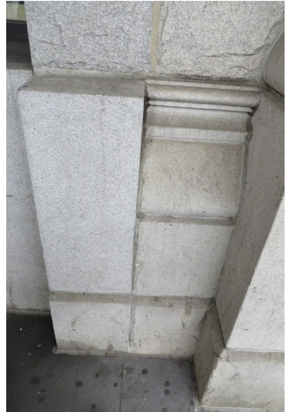
MODIFIED BASE - ORIGINAL DETAIL PARTIALLY REPLACED
