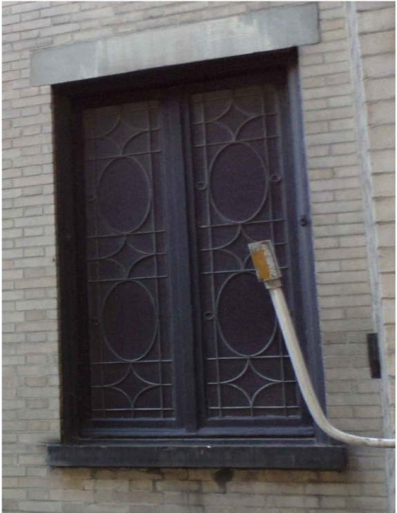
EXISTING WINDOW CONDITION - EXTERIOR VIEW
