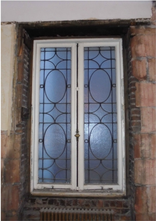
EXISTING WINDOW CONDITION - INTERIOR VIEW
