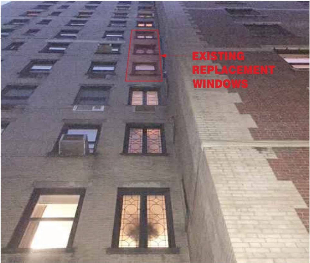
Existing Partial Building West Facade Courtyard
