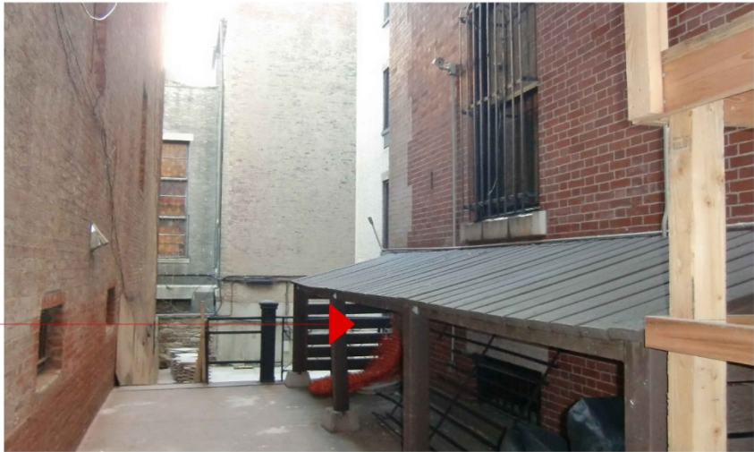
West Facade Courtyard Corridor at Service Area
