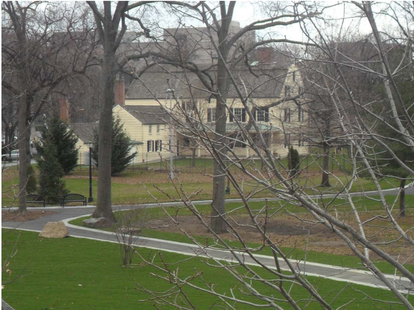
1 - View to back porch of Manor House
