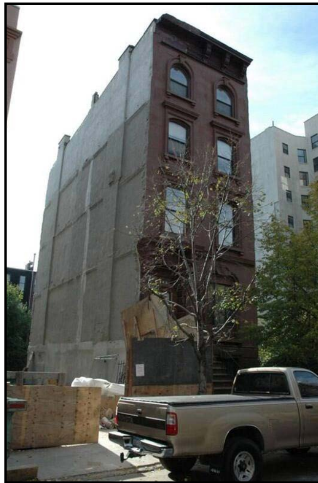
110 W 123 STREET PRIOR TO DEMOLISHING 5 STORY (APPROXIMATELY 60 FT IN HEIGHT)
