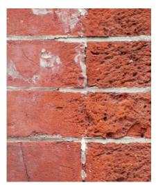
The negative effects of abrasive cleaning or sand blasting on brick (shown on right).
