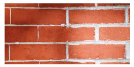
In a good repointing job (left), the new mortar matches the existing mortar in color, hardness, and joint profile. A poor repointing job (right) can destroy the original appearance of the building. Here, the mortar joints are too wide and the composition of the mortar is too hard.
