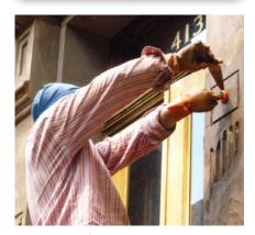
A brownstone facade being partially resurfaced with matching stucco.
