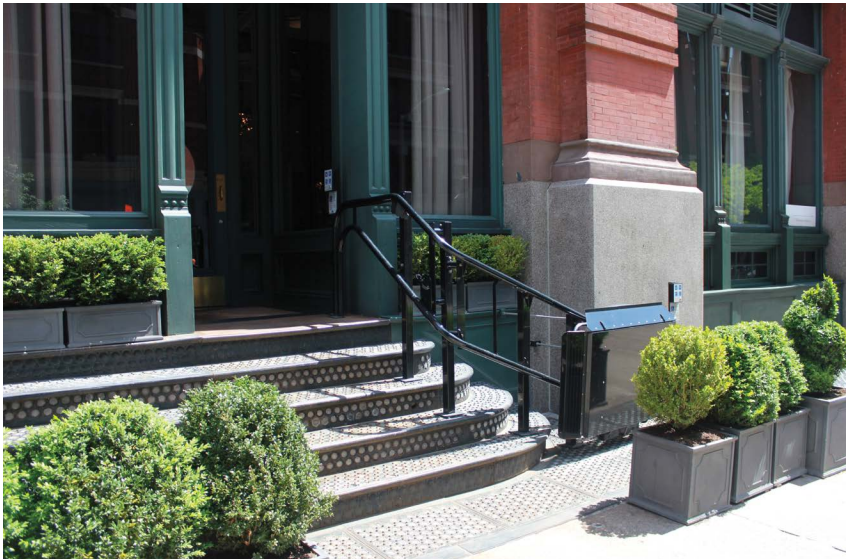
A chair lift on rails, finished to match the existing metal stairs and installed with minimal attachment points.
