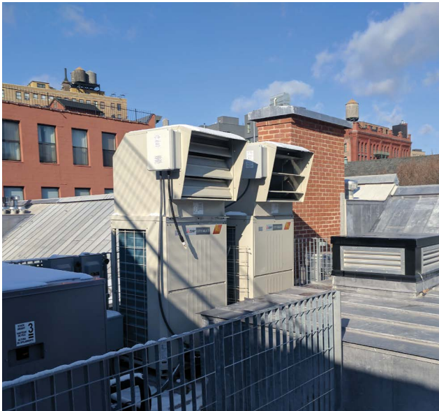
Rooftop HVAC installations, including vents and condensing units, can be minimally visible if it is not possible to make them non-visible from public thoroughfares.
