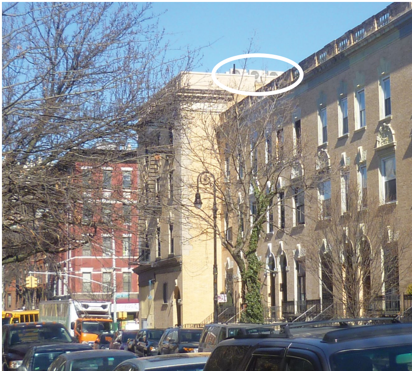
Minimally visible rooftop HVAC units, as seen from a public thoroughfare.
