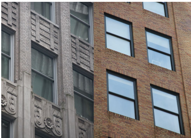
Through-wall HVAC installations should not be installed at decorative masonry (at left), but may be installed at plain masonry (at right).
