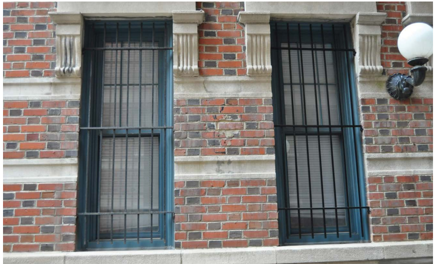
Security grilles attached at limited points to window surrounds at the ground floor.
