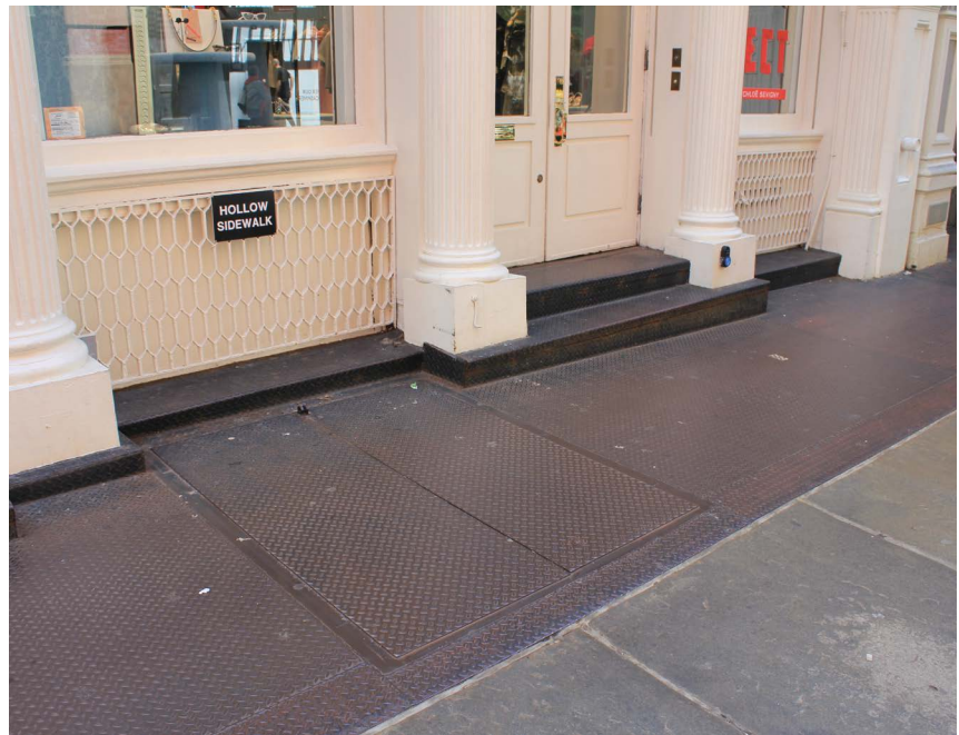
Deteriorated historic vault lights can be covered and protected by steel diamond plate with a dark painted finish, as seen here.
