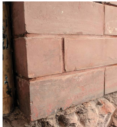
The mortar joints have been repointed to match the historic joints in terms of color, texture, and profile.
