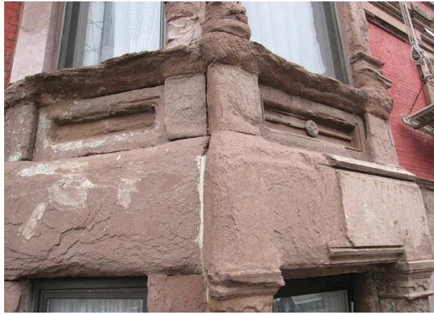
Significantly deteriorated brownstone, often referred to as delamination.
