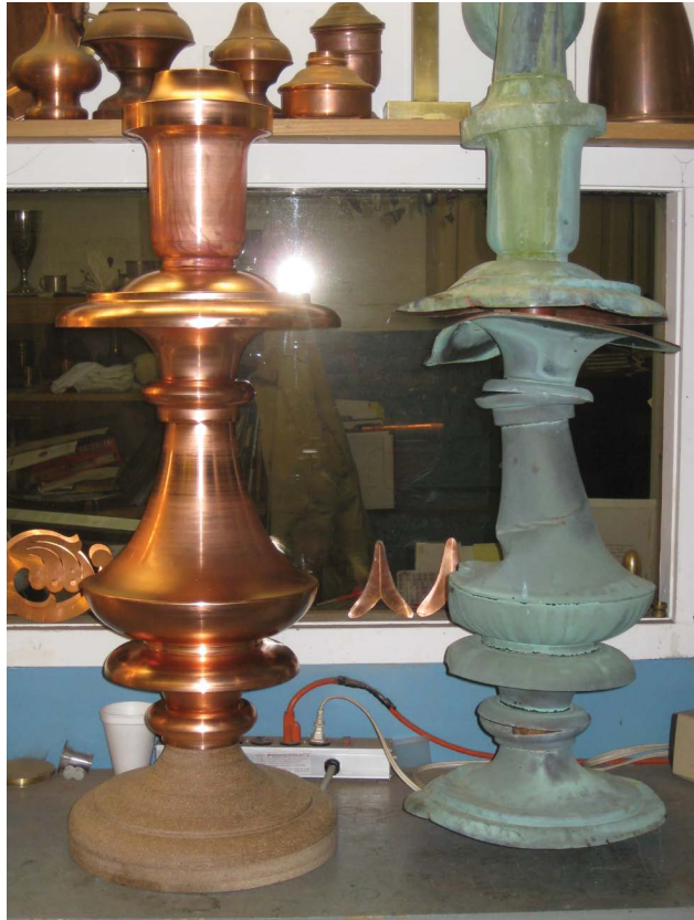
Replacement decorative metal feature matches the historic metalwork.
