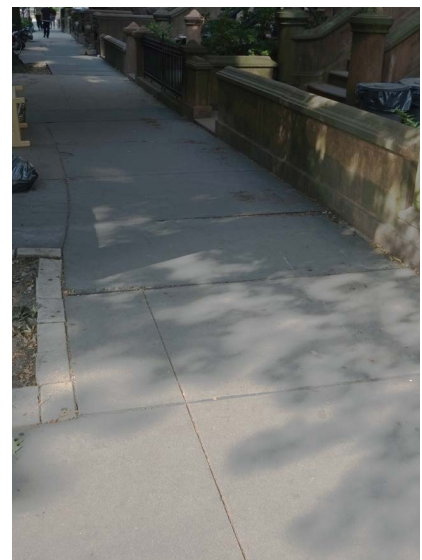
A new concrete sidewalk with saw-cut joints, tinted to match the adjacent historic bluestone.
