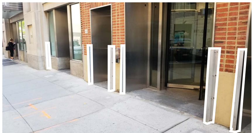
Posts for removable flood protection barriers, all with a neutral finish, installed at plain masonry at select openings.
