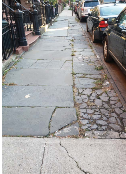
Heavily damaged or crushed bluestone pavers can be removed and replaced with new bluestone or tinted concrete to match.
