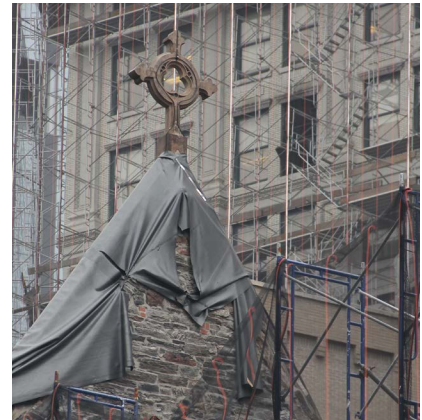
Fragile or deteriorated architectural features can be stabilized and protected in place, as seen here while construction is in progress.
