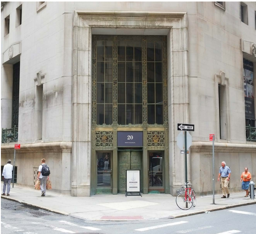
Special window featuring densely gridded multi-light and curved glass sashes with stained glass transoms.
