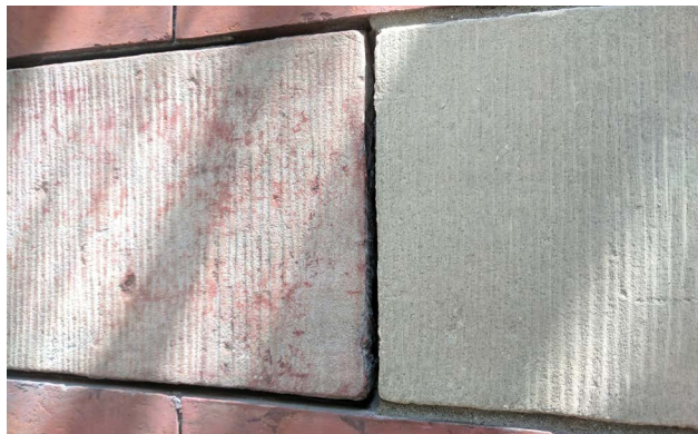
The color of the historic masonry on the left is matched by the mineral stain coating on the right.
