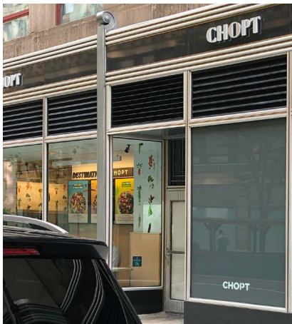
An example of grey-scale translucent film installed to hide a kitchen space at the interior.
