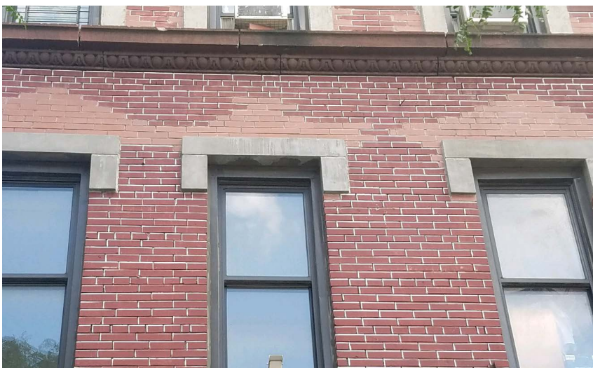
Example of a poor brick match. Note how the new bricks (above the lintels) do not match the historic bricks, calling undue attention to the repair.
