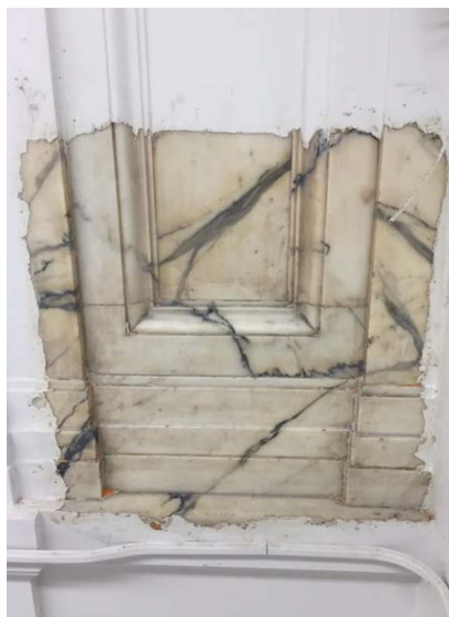
Coating removal without damaging the historic material
