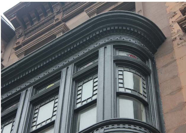
Special window featuring densely gridded multi-light and curved glass sashes with stained glass transoms.
