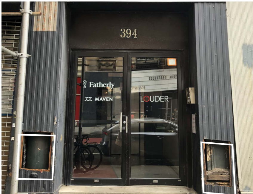
The historic storefront has been covered with metal cladding. Probes have revealed the original cast iron piers.
