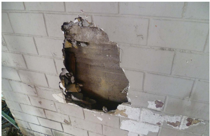
Example of a major investigative probe that would require a permit.
