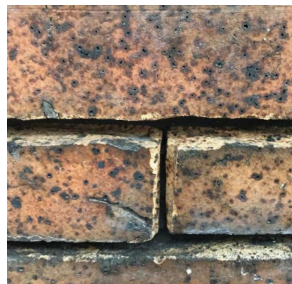
Inappropriate mortar joint removal. Note how the edges of the bricks have been damaged by the process.
