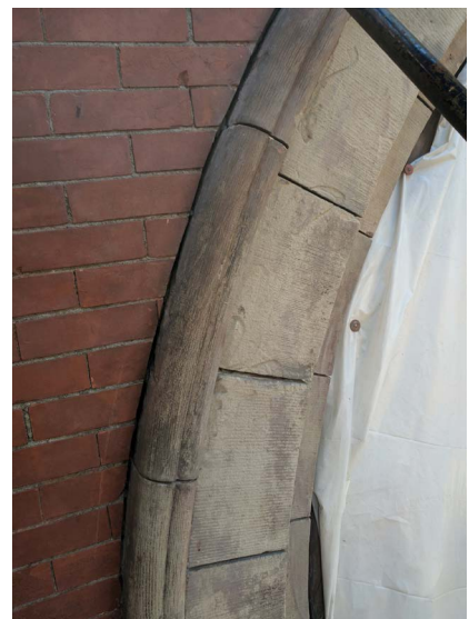
Historic masonry damaged by harsh coating removal and cleaning methods
