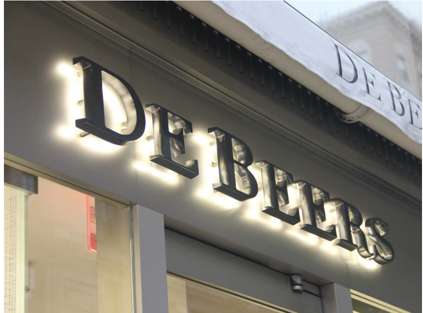
Halo-lit, pin-mounted lettering at a signband.
