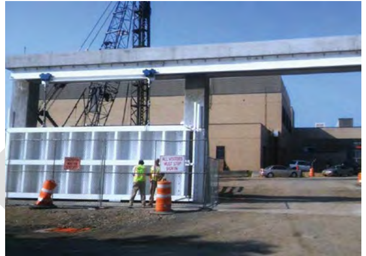
Figure 8: Over-head trolley roller gate at Bay Park WWTP.
