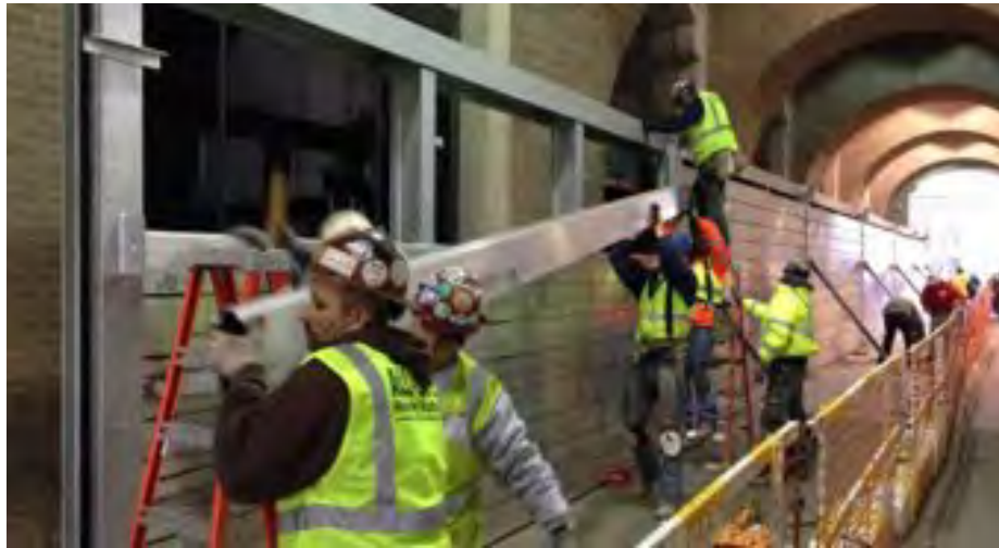
Figure 5: Plank-type system installed at Verizon Telecommunications, 140 West Street, NYC
