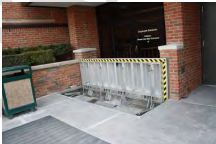
Figure 6: Activated flip-up barrier protecting entranceway. (Source: PS Flood Barriers)
