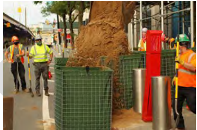
Figure 4: Filling metal-reinforced containers (HESCO Barriers) with dirt in preparation for Tropical Storm Isaias near South Street in Lower Manhattan. (Source: G.N.Miller/NYPost)
