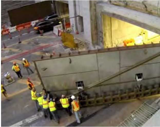
Figure 7: Swing-hinged gate at Hugh L. Carey tunnel entrance
