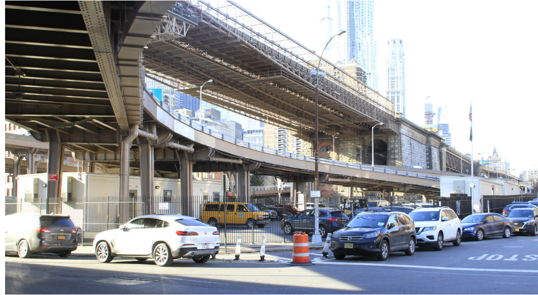
2. VIEW LOOKING NORTH FROM SOUTH STREET
