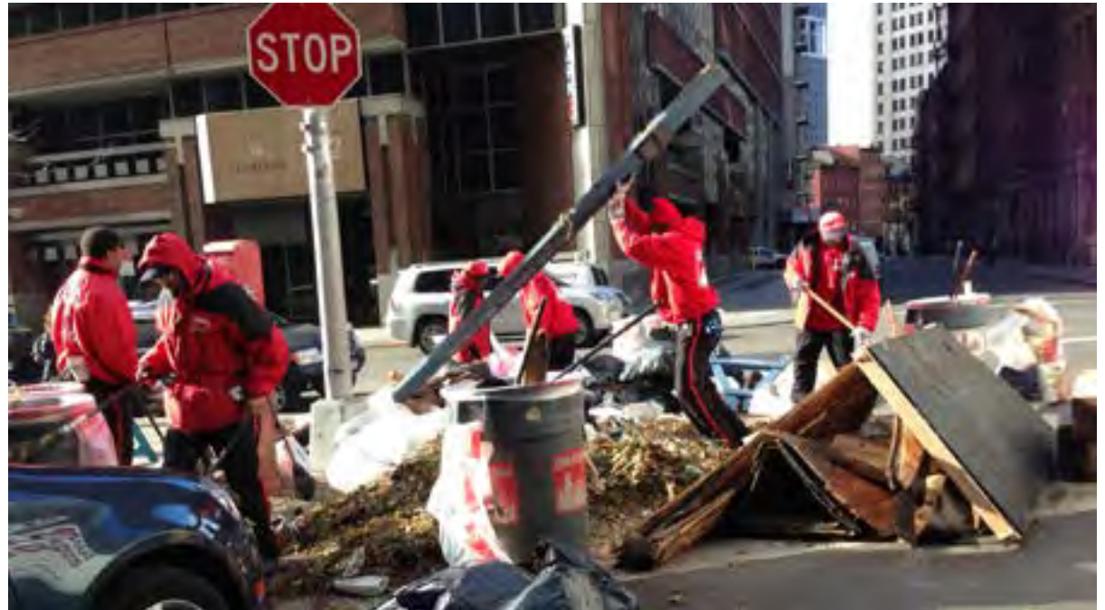
Businesses, organizations, and governmental entities immediately got to work to repair streets and infrastructure in Sandy's wake. Source: Courtesy of the Alliance for Downtown New York.
