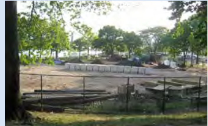
Current site conditions at East River Park. Source: Courtesy of LES Ecology Center.
