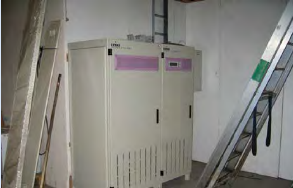
This project may provide funding for measures such as the installation of fixed backup generators, to supply power in the event of an outage. Source: Flickr user Jemimus (Robert), licensed under Creative Commons.
