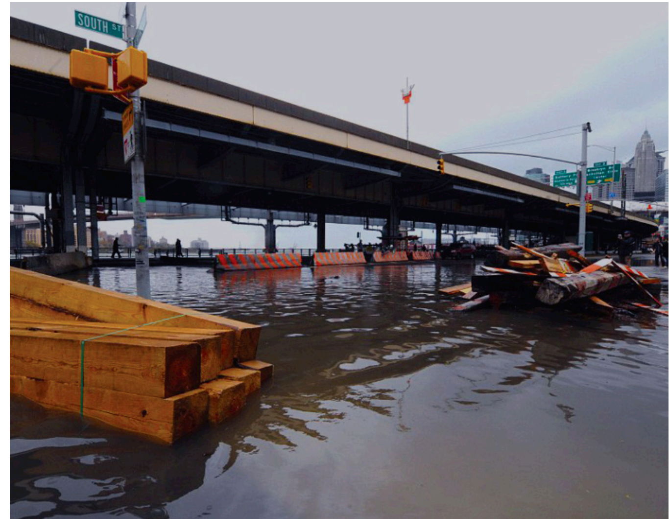
South Street Post-Hurricane Sandy
