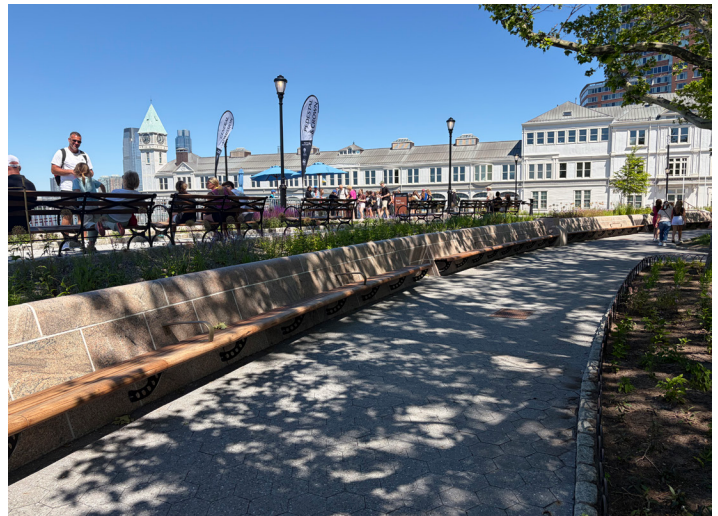
View of Completed Park Promenade facing Pier A Building
