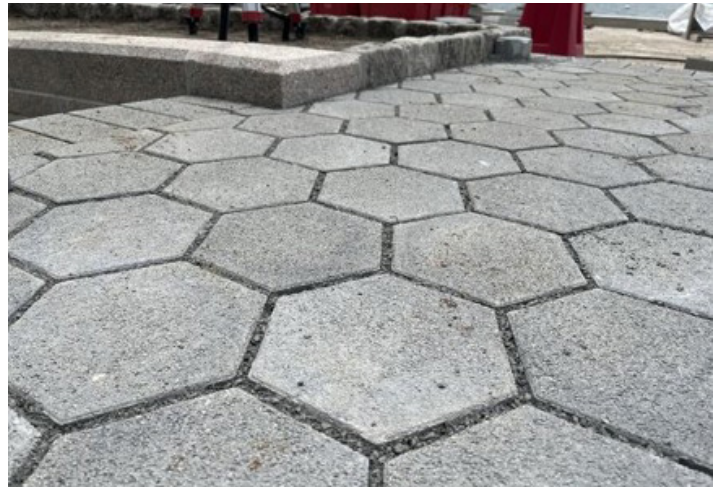
Image: Permeable hex pavers designed to capture storm water and reduce runoff.
