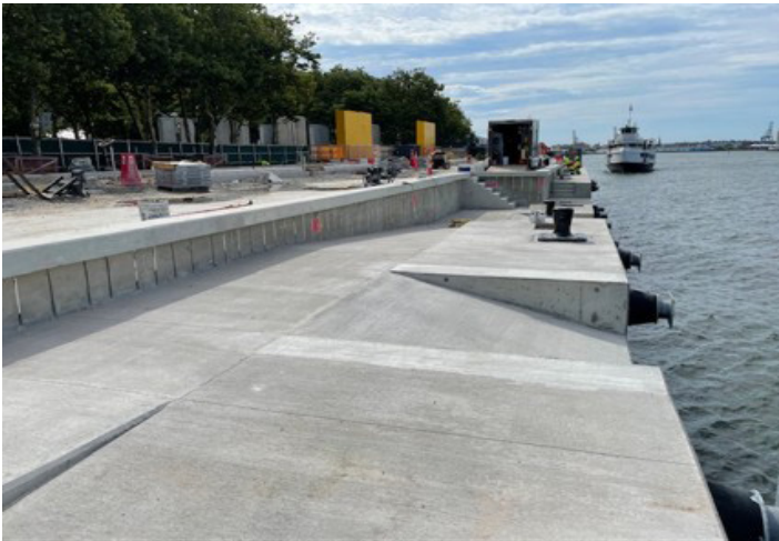
Image: Completed concrete of Slip 3 with associated marine appurtenances. Installation of the fendering has begun along wharf face.
