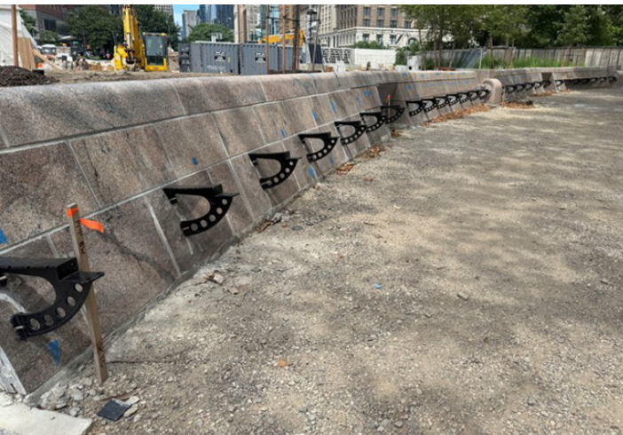
Image: Granite backed bench wall with metal brackets; wooden benches and bronze armrests forthcoming.
