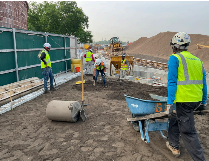
Image: Planting soil is spread and compacted to optimal conditions to facilitate future plant growth; the density and infiltration rate of soil is verified via field tests.
