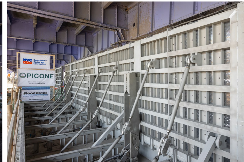
Flip up gate in open position – March 2025
