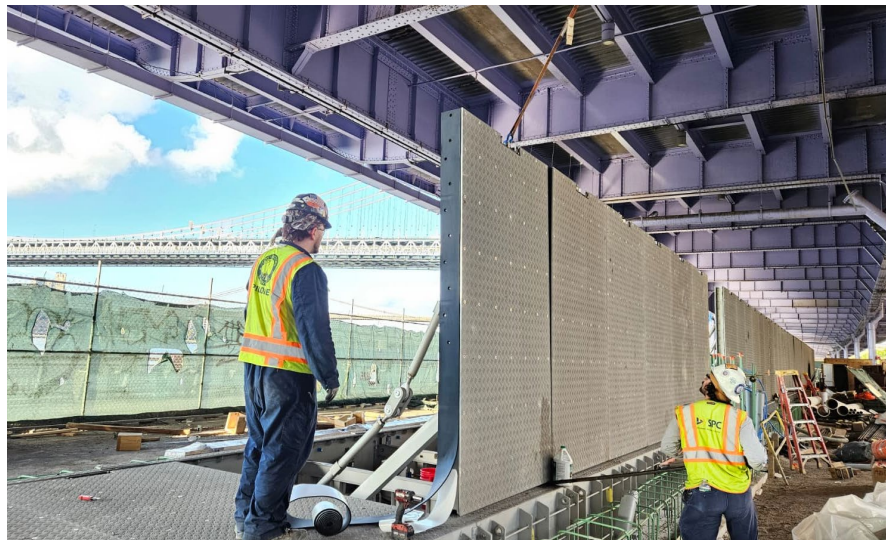
Flip up gate installation – September 2025
