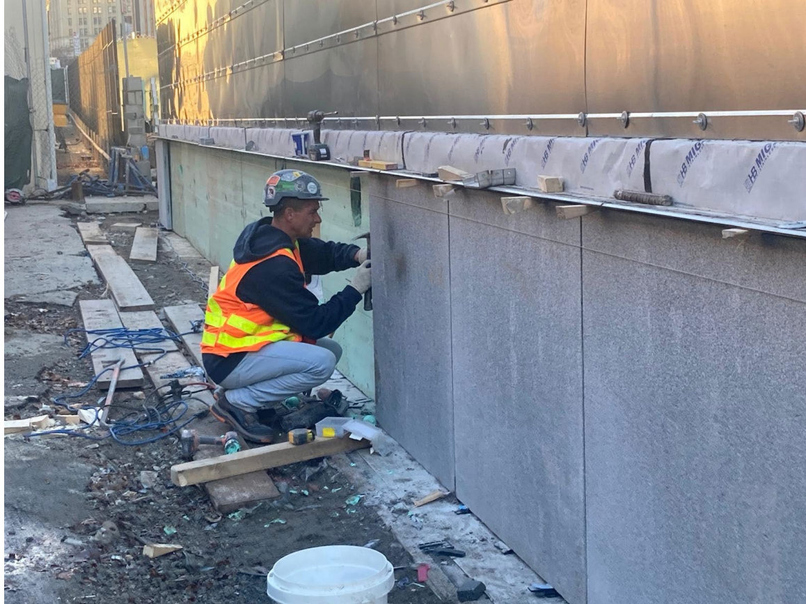
Installation of granite cladding on Interceptor Gate Building – March 2026
