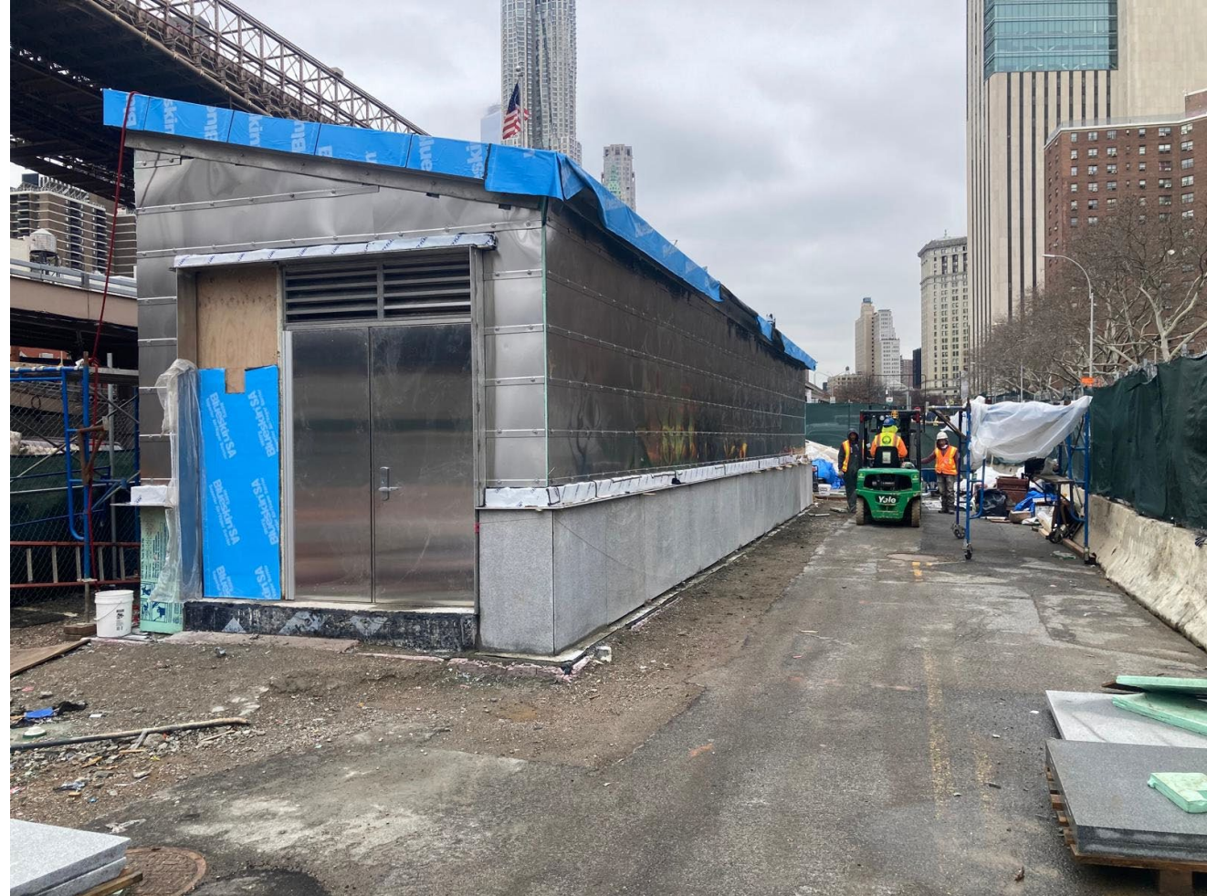
Construction of Interceptor Gate Building – March 2026
