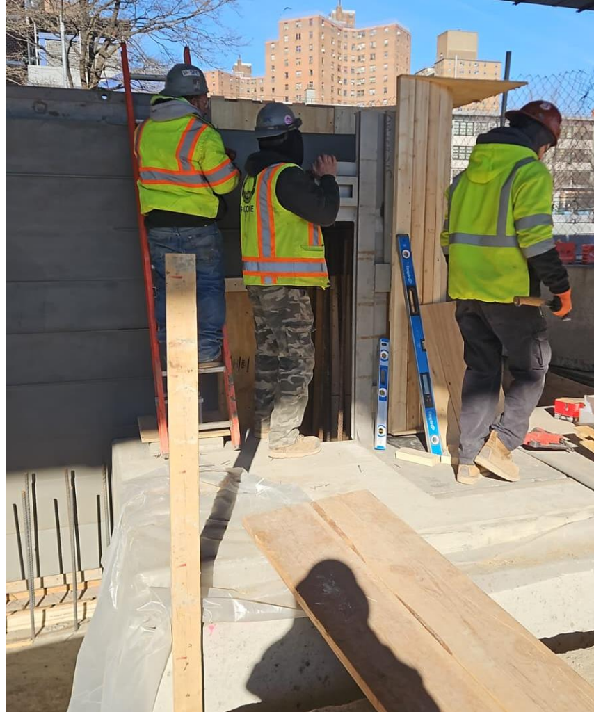
Formwork for independent floodwall under FDR Drive near Montgomery Street – January 2026
