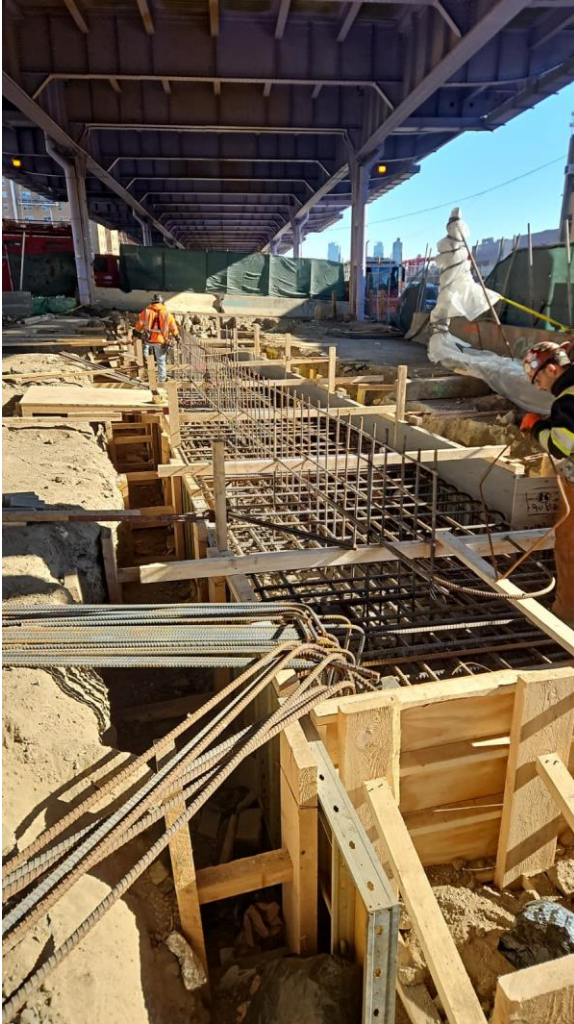
Formwork for floodwall footing under FDR Drive near Montgomery Street – January 2026
