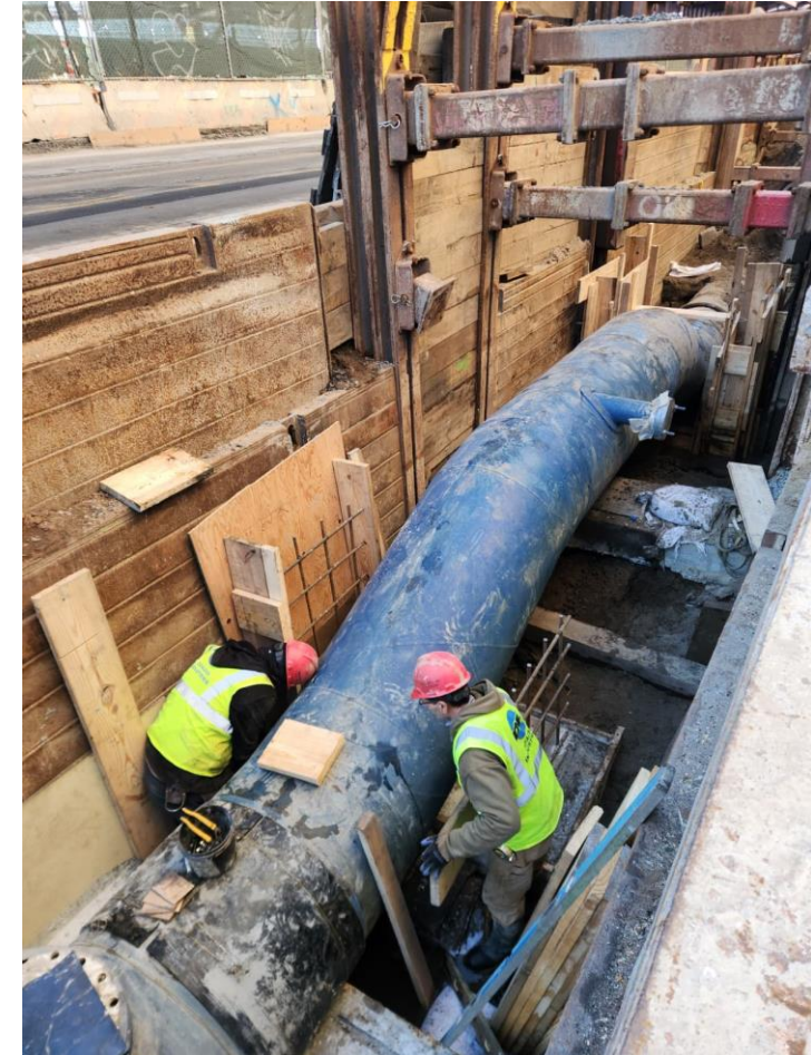
Trunk main installation in South Street – January 2026
