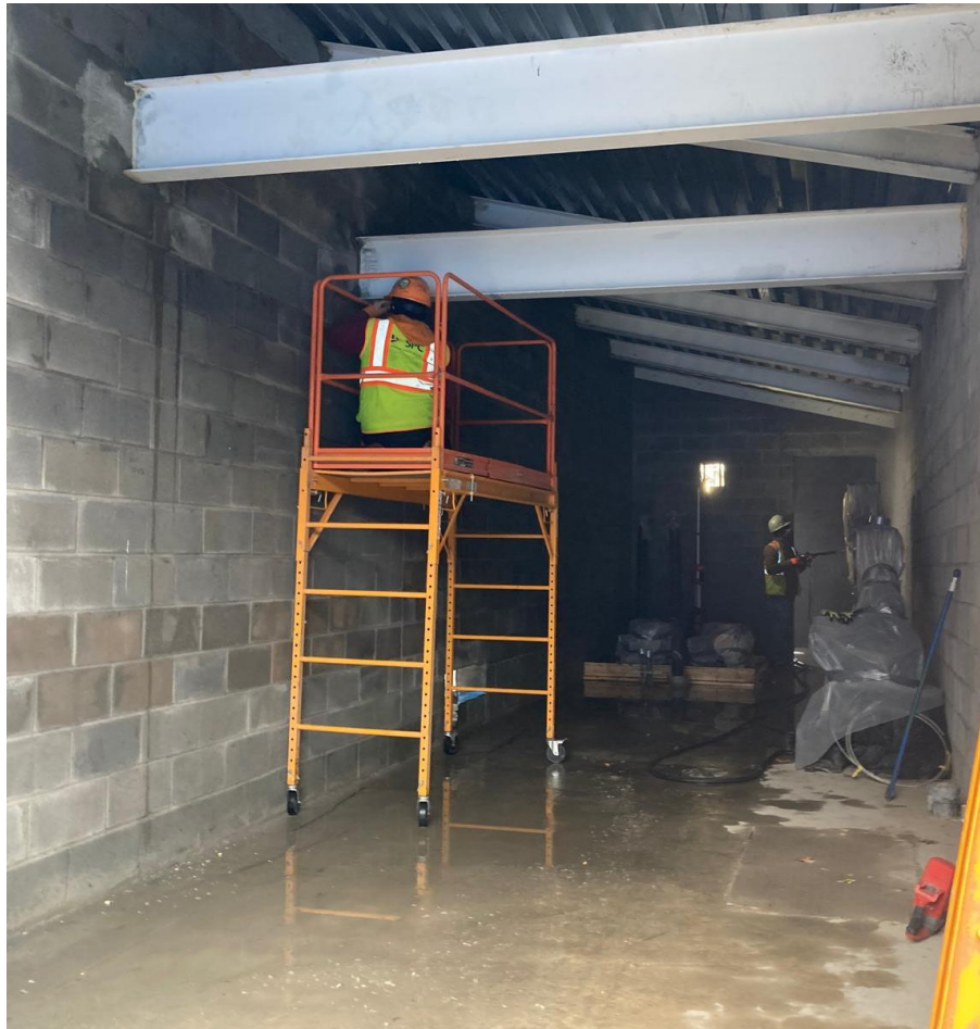
Work on interior of interceptor gate building – January 2026
