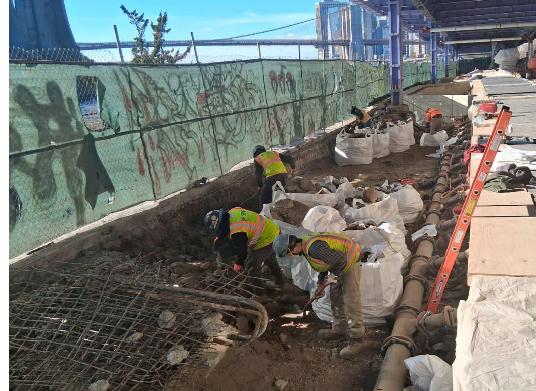
Excavating for landscape features on the esplanade – January 2026
