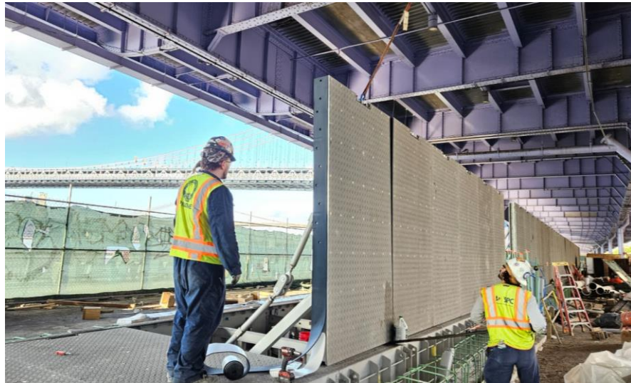
Flip up gate installation – September 2025
