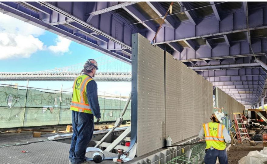
Flip up gate installation – September 2025
