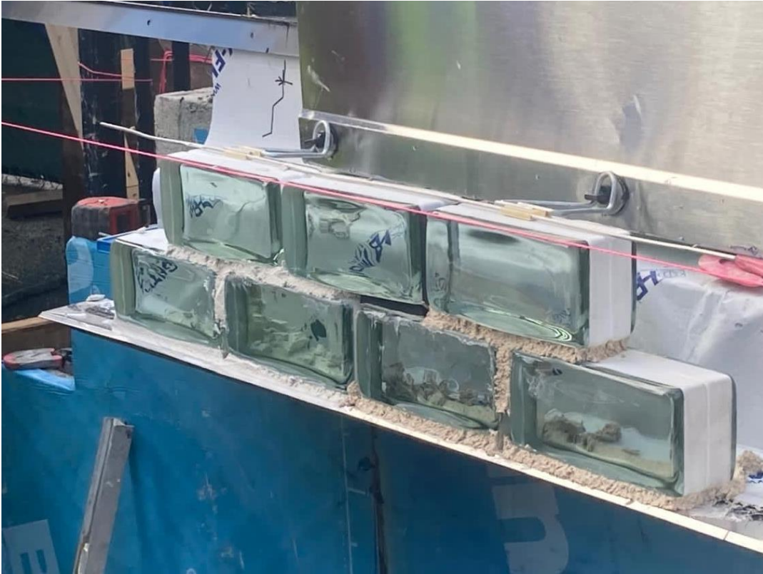
Interceptor Gate Building glass brick mockup – October 2025
