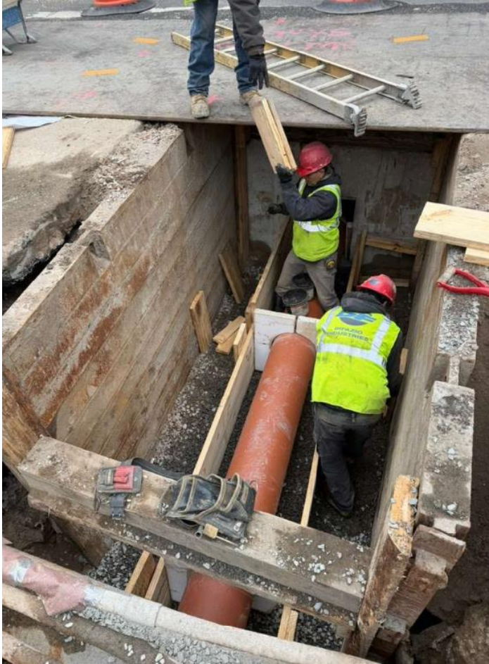
Installation of 12-inch sewer pipe at South Street and Catherine Slip – November 2025
