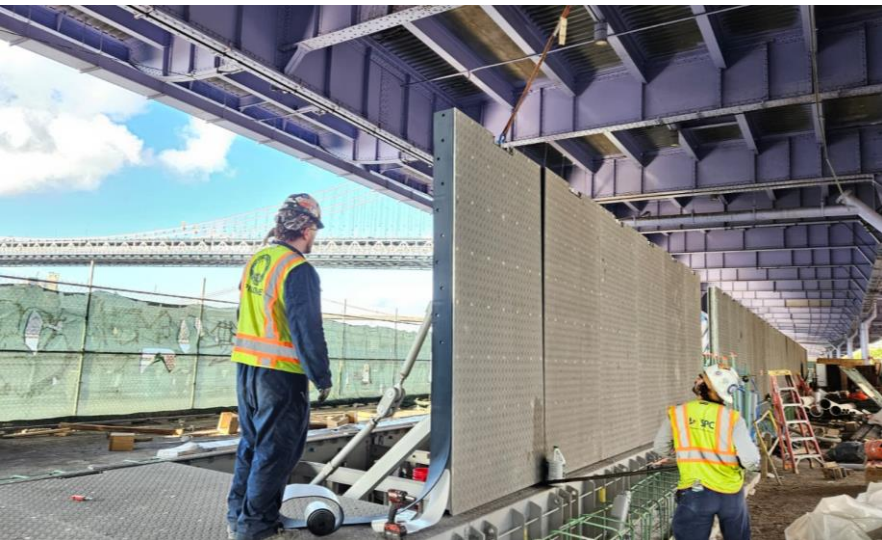
Flip up gate installation – September 2025
