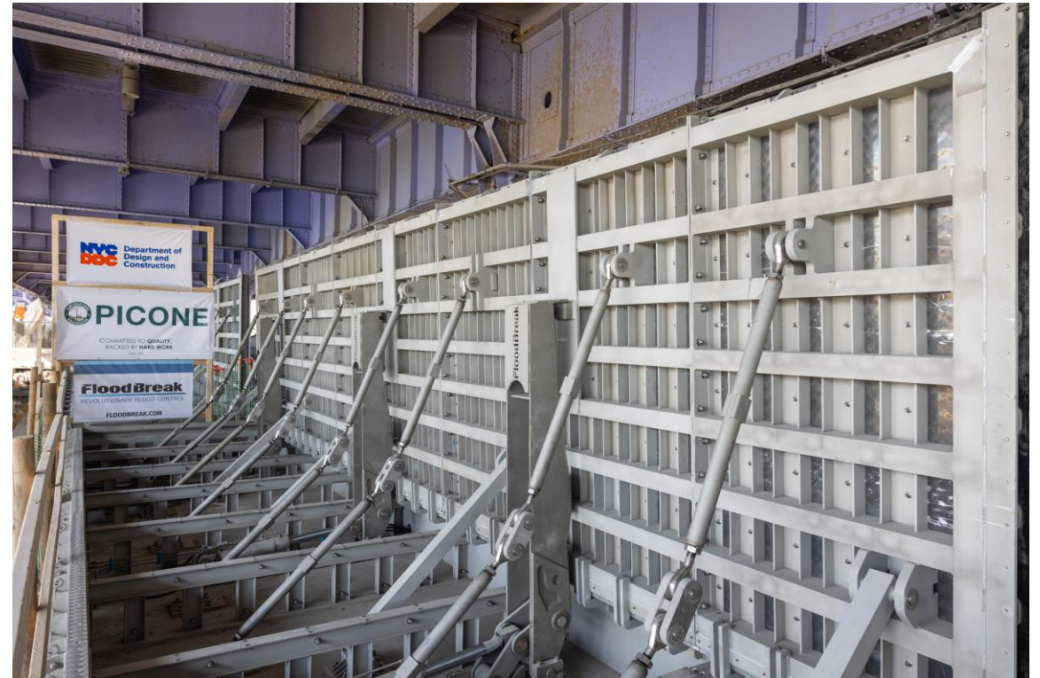
Flip up gate in open position – March 2025
