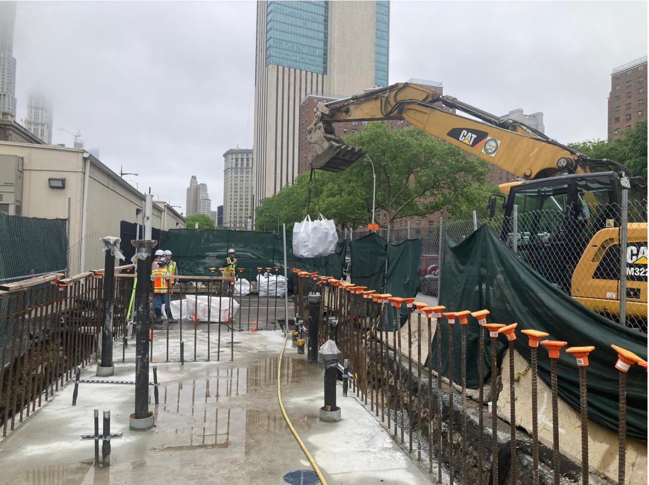
Interceptor Gate Building foundation installed, utility installations – May 2025
