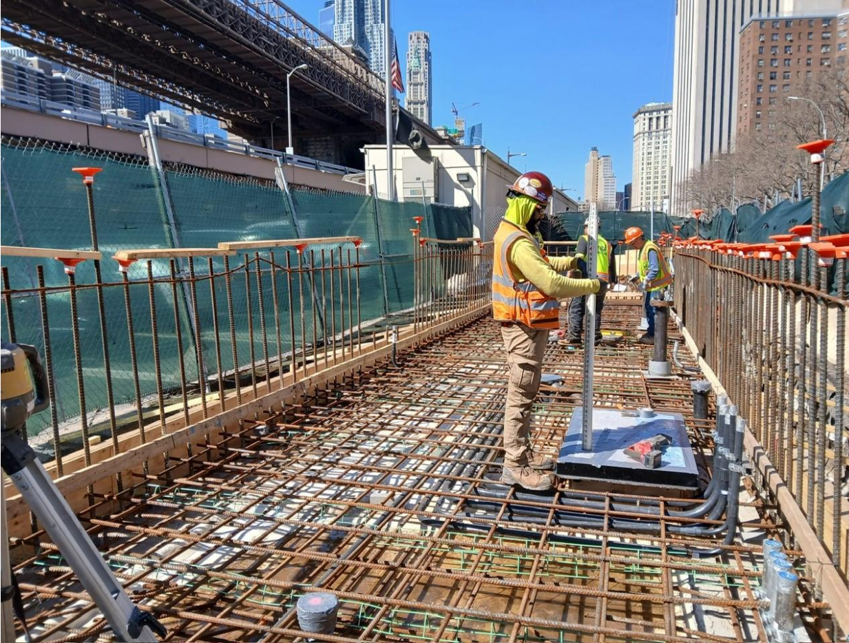
Prepping to pour concrete slab for Interceptor Gate Building – March 2025
