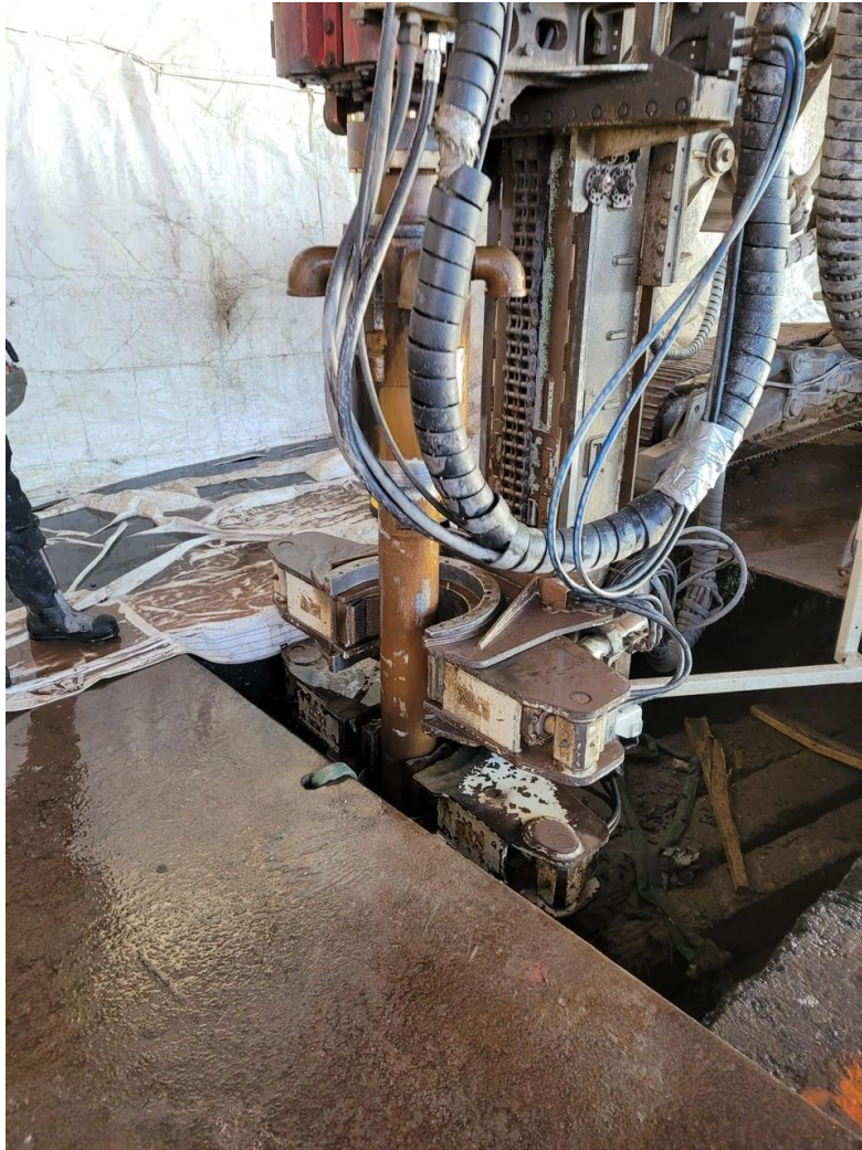
Drilling for pile installation – March 2025
