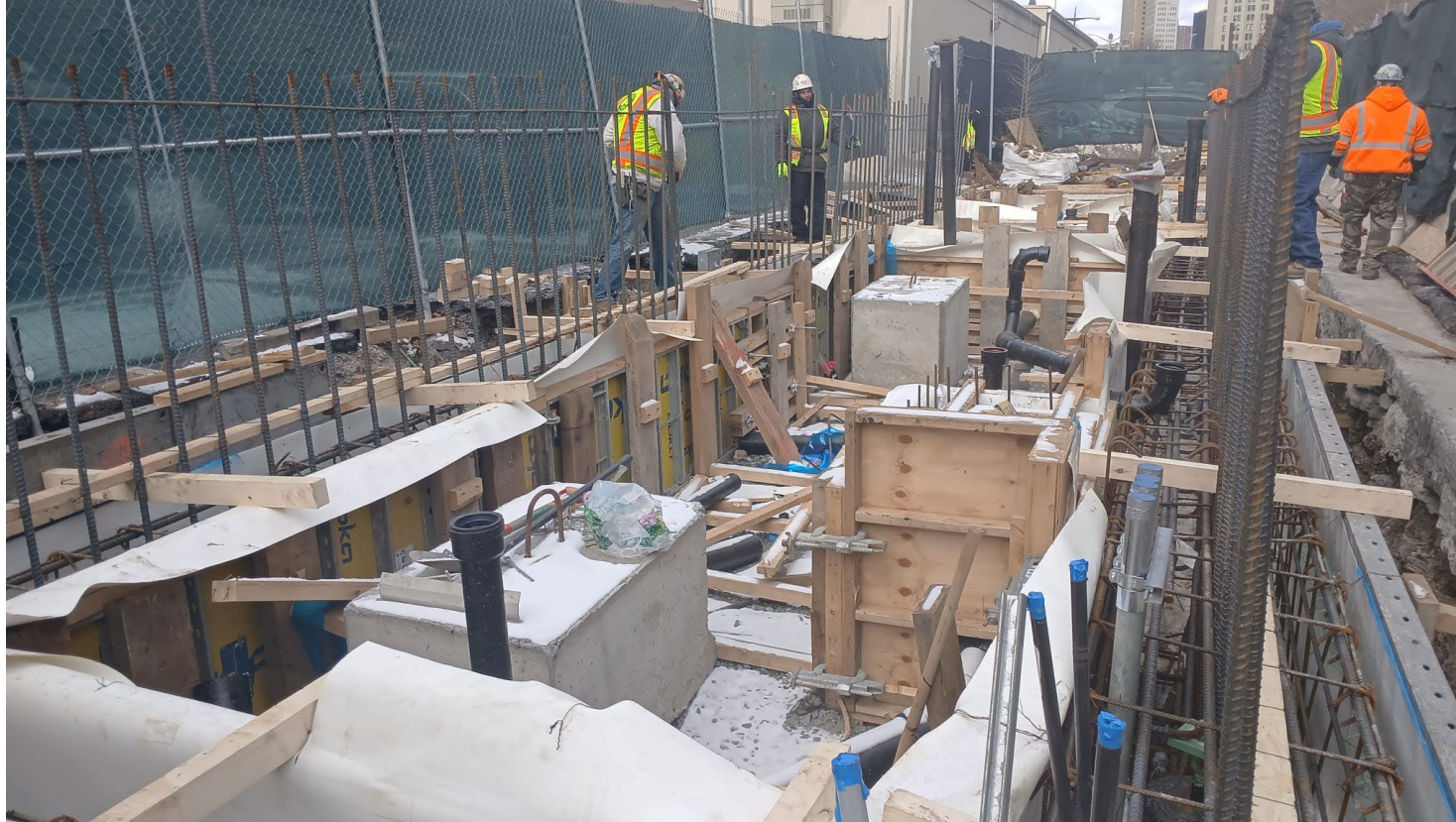
Rebar installation for foundation of Interceptor Gate Building – January 2025
