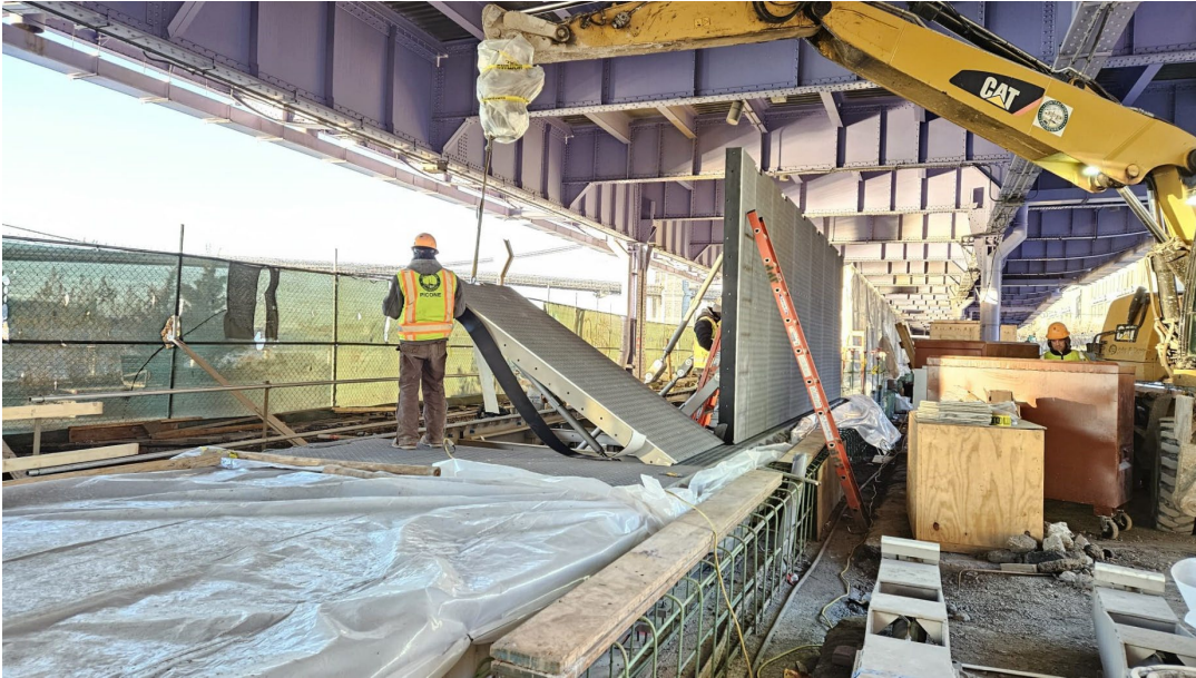
Flip up gates being installed – January 2025
