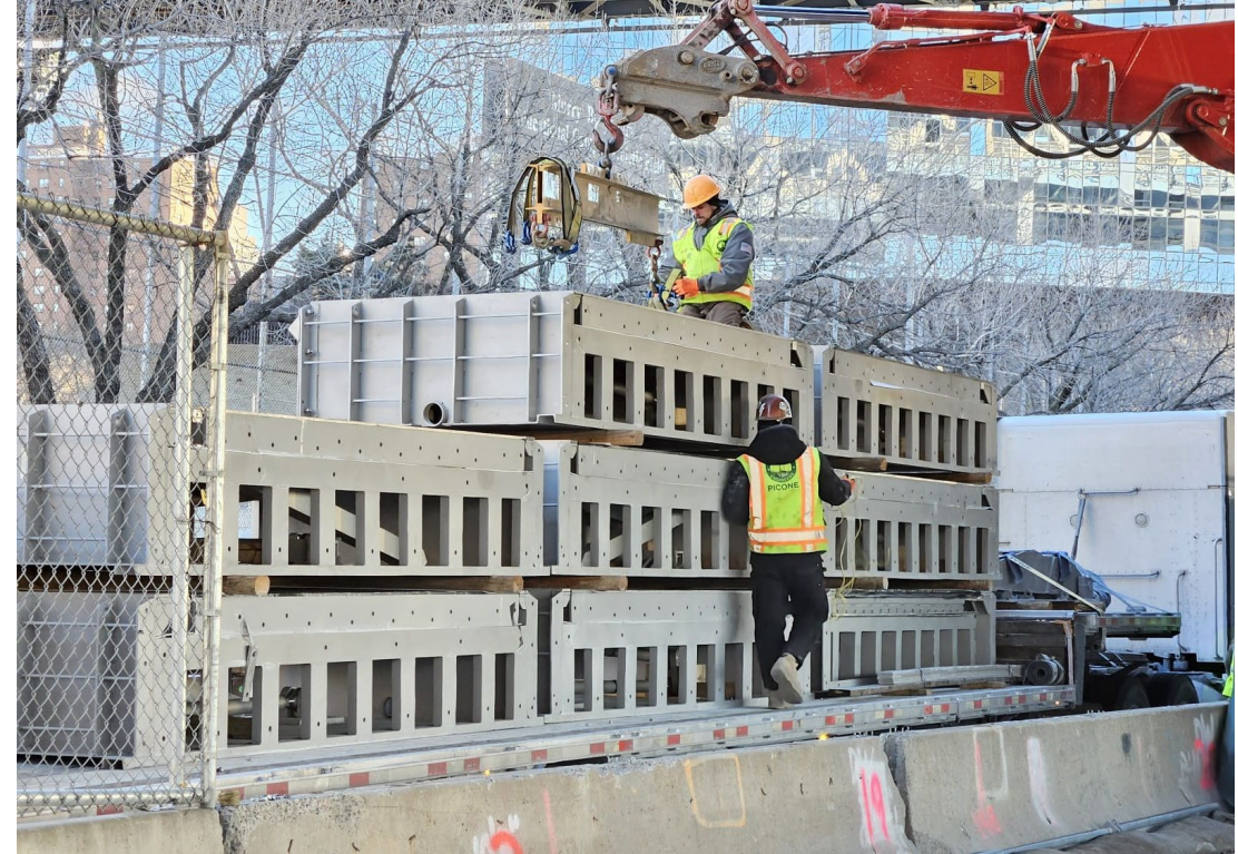
Flip up gate segments delivered to site – January 2025
