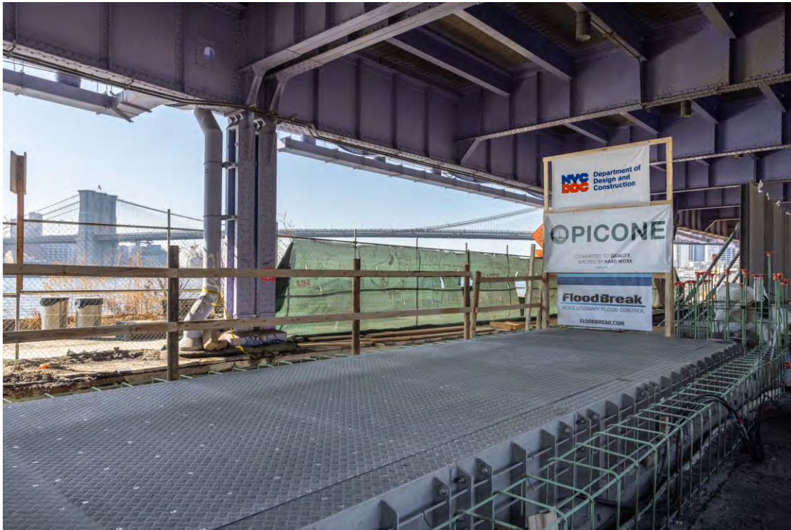
Flip up gate in closed position – March 2025
