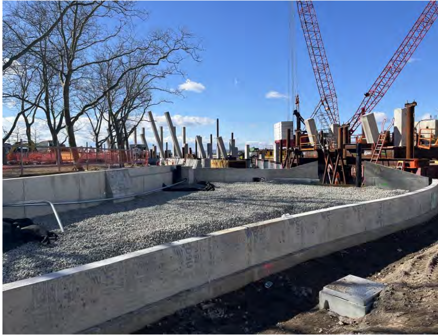
February 2025 – Placement of Ultra Lightweight Foam Glass Aggregate Fill
