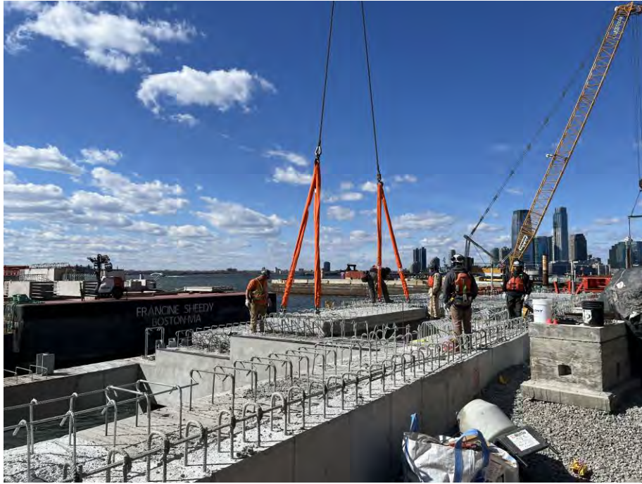
February 2025 – Precast Plank Installation
