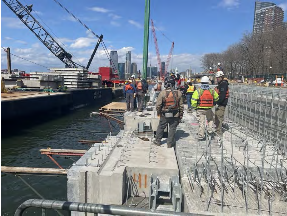
April 2025 – Deck Reinforcement & Fascia Panels
