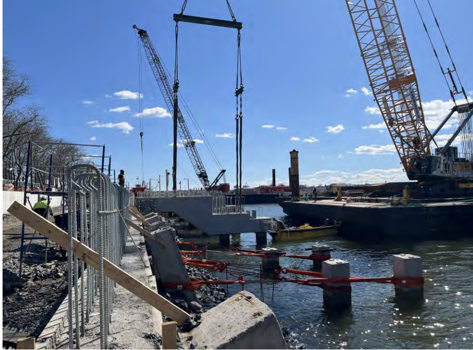
December 2024 – Installation of Precast Pile Caps
