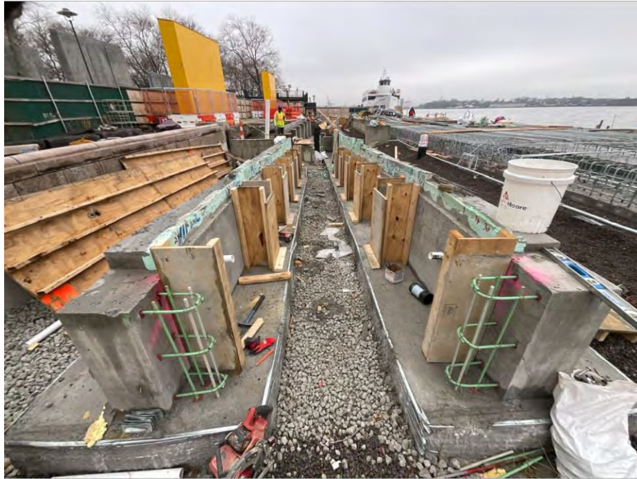
March 2025 – Foundations for Gardens of Remembrance Ramps
