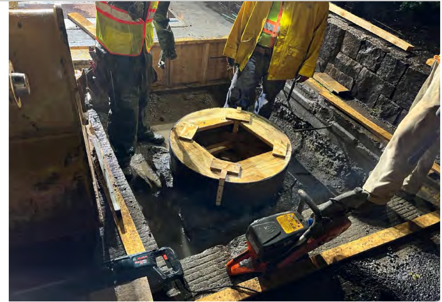
Tide Gate Chamber installation in Pier A Plaza, and watertight manhole cover installation
