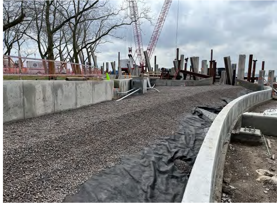
March 2025 – Placement of Expanded Shale Clay & Slate Fill
