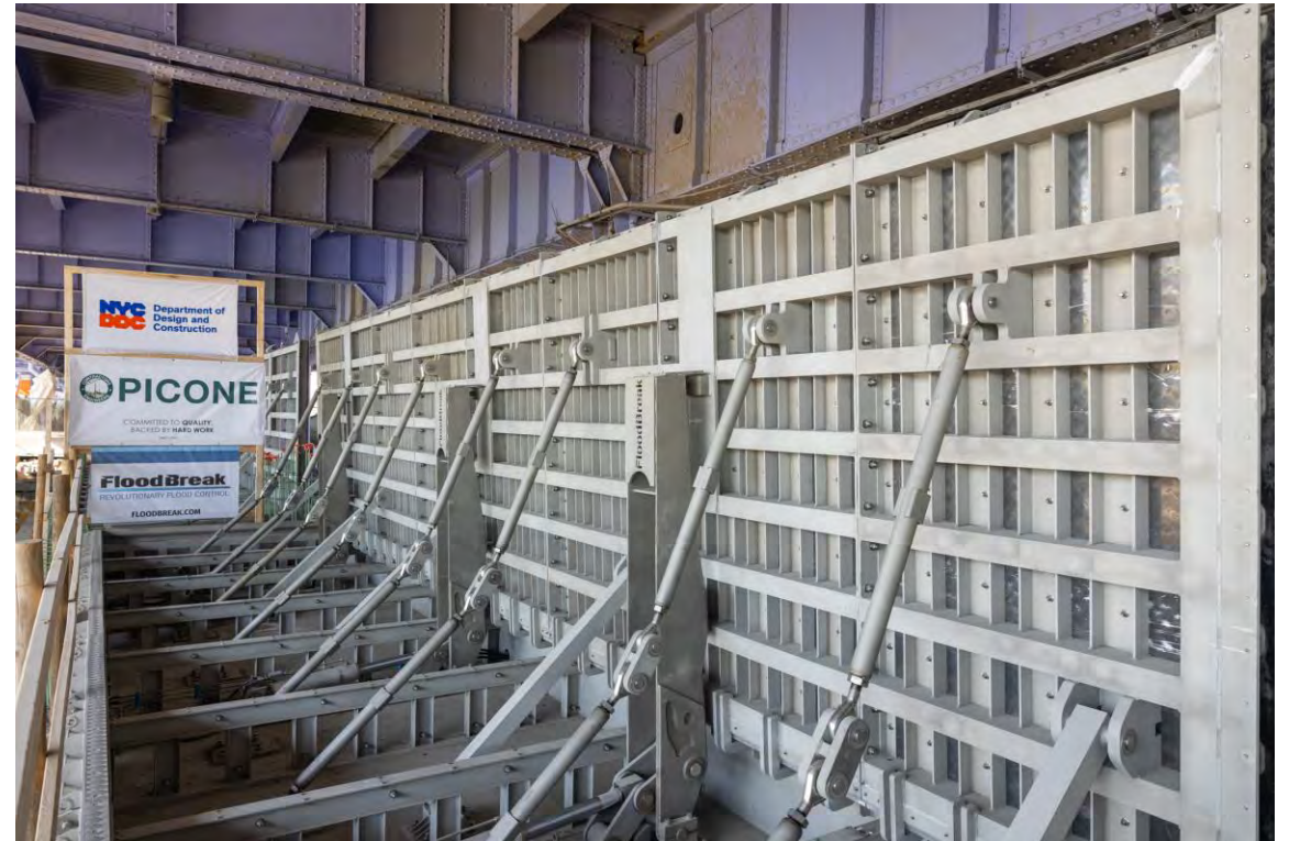
Flip up gate in open position – March 2025
