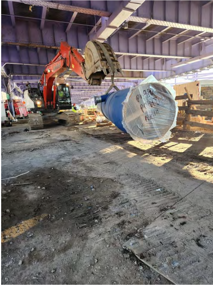
Trunk water main installation under FDR Drive – February 2025
