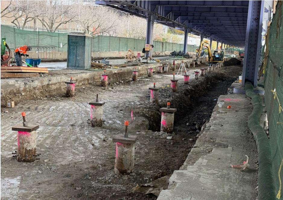
Micro-piles for floodgate foundation – October 2024
