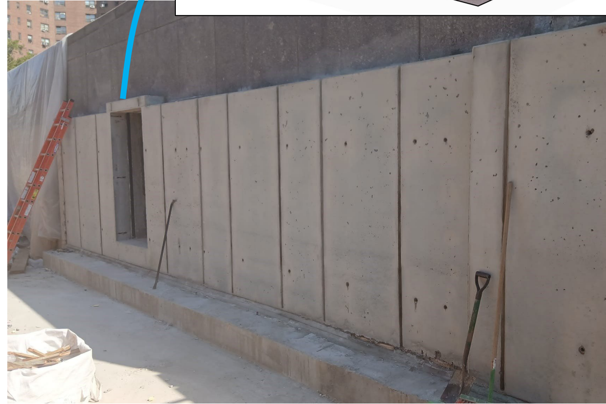
Floodwall tie-in to FDR Drive off-ramp – September 2024
