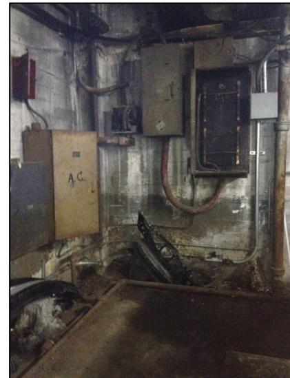
Photograph 8: Decommissioned electric panels and debris at 143 West 108<sup>th</sup> Street.
