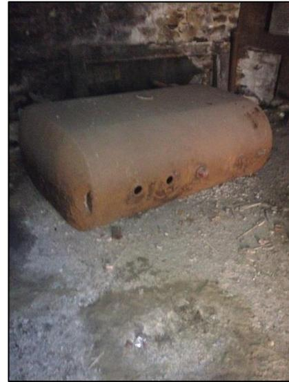
Photograph 2: Defunct 275-gallon AST in partial basement of 103-107 West 108<sup>th</sup> Street.
