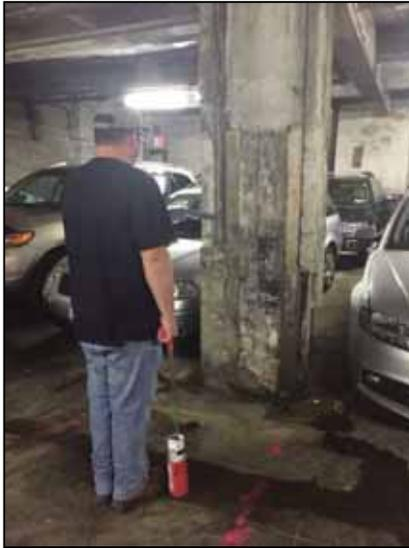
**Photograph 1.** Geophysical surveyor marking out identified utilities in the basement of 151-159 West 108<sup>th</sup> Street.
