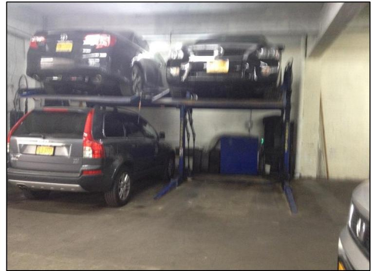
Photograph 6: Above ground hydraulic lifts at 143 West 108<sup>th</sup> Street.
