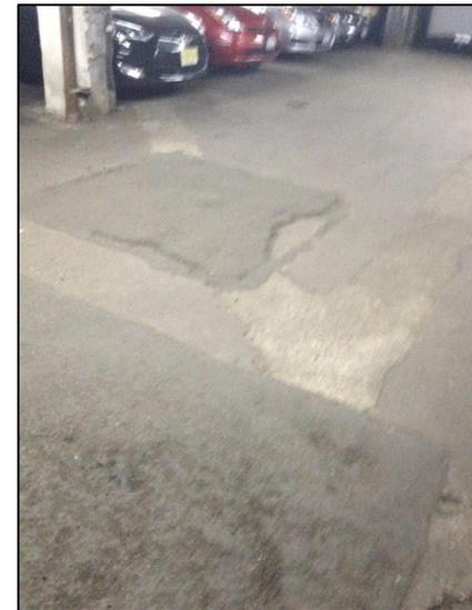
Photograph 16: Patched concrete floor in basement of 151-159 West 108<sup>th</sup> Street.
