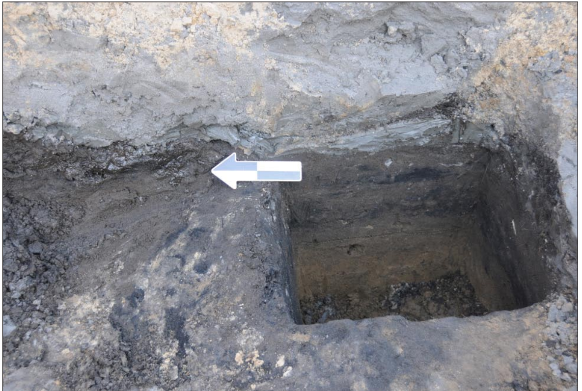
Facing east showing east wall of Test Pit 8.1 on the floor of Trench 8 at a depth of 12 feet below ground surface. 12 Original ground surface has been disturbed and smelled strongly of petroleum
