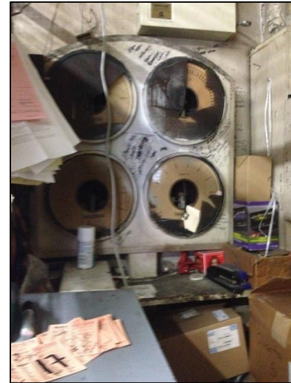
Photograph 14: Decommissioned meters for four USTs at 151-159 West 108 th Street.
