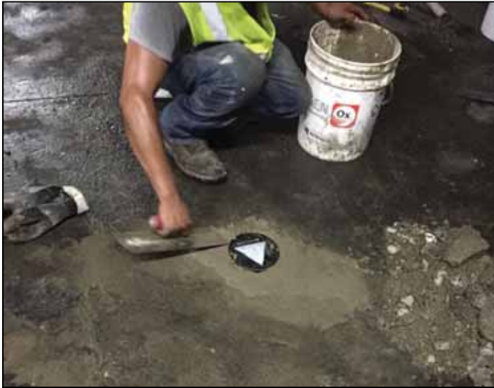
Photograph 5. Completing the concrete pad and manhole for a permanent groundwater monitoring well.
