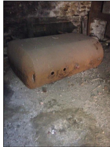
Photograph 2: Defunct 275-gallon AST in partial basement of 103-107 West 108 th Street.
