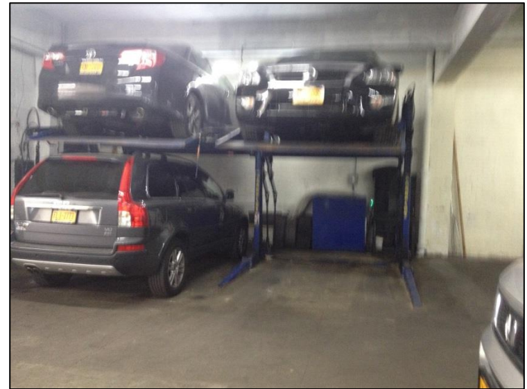
Photograph 6: Above ground hydraulic lifts at 143 West 108 th Street.
