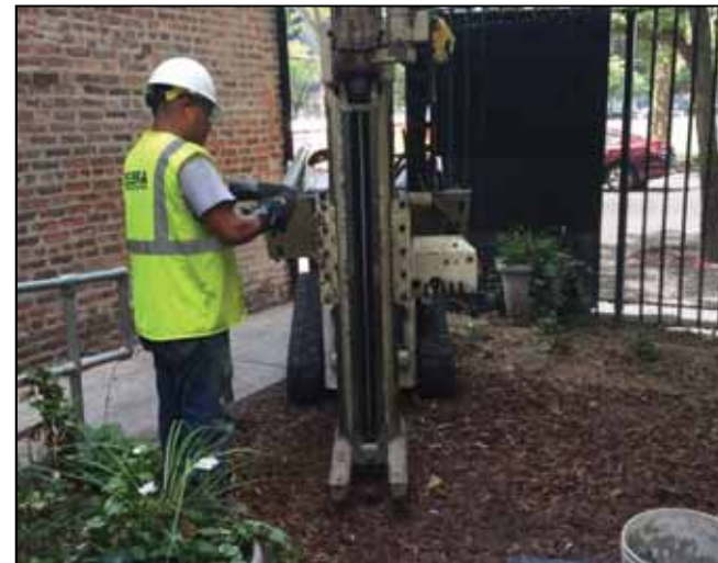
Photograph 8. Limited access retrofitted track-mounted direct-push probe unit advancing soil boring in the garden area of 145-149 West 108 th Street.
