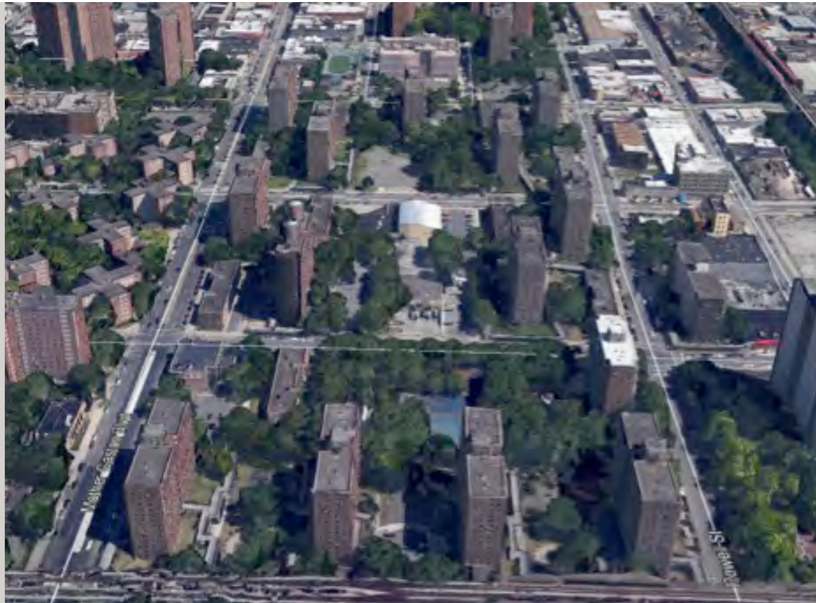
Above, an aerial view of the Van Dyke Houses.
