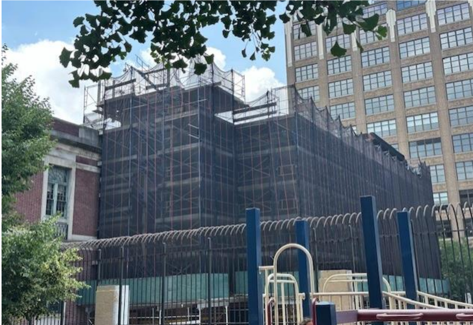
Extensive scaffolding is supporting building's west façade adjacent to outdoor pool; view from playground in J.J. Walker Park, June 2024
