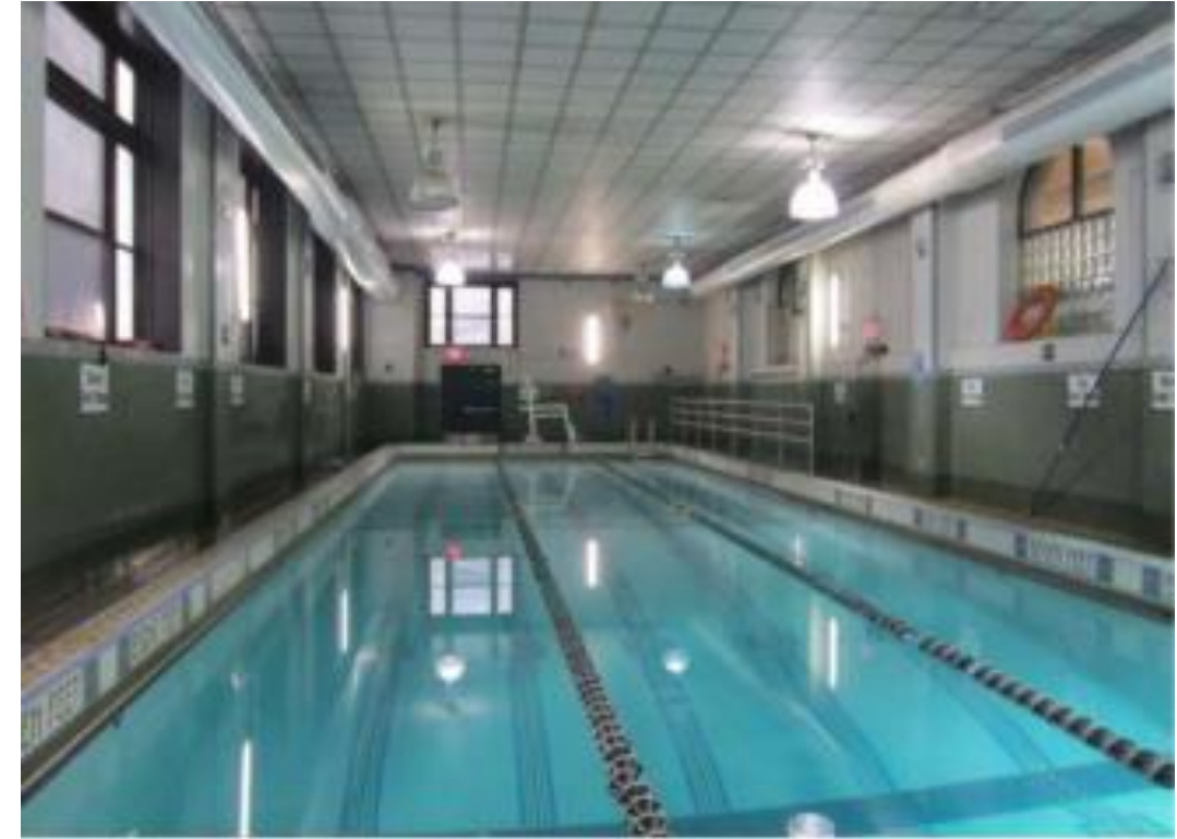
None code-compliant indoor pool has virtually no pool deck. Renovation of building would need to bring pool up to code and install pool decks, reducing size of pool basin.
