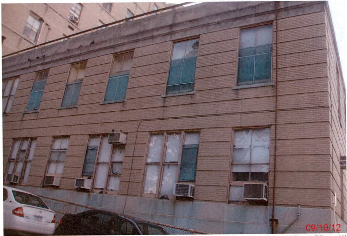
Southwest Rear View (1)
