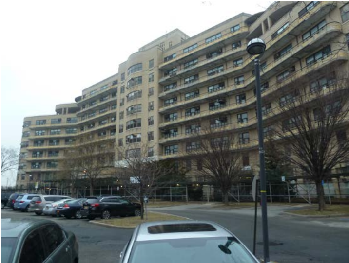
1. Southwestern façade of the T Building.
