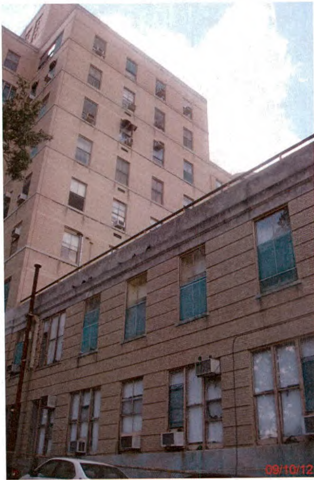
Southwest Rear View (2)
