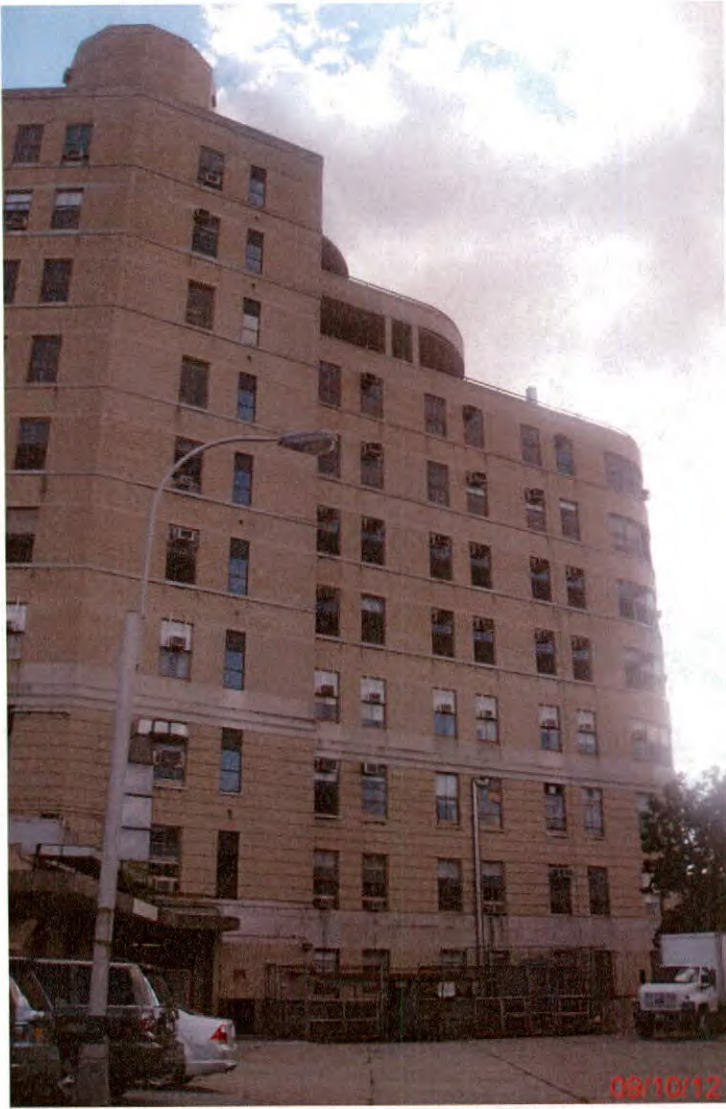
Southwest Rear View (5)
