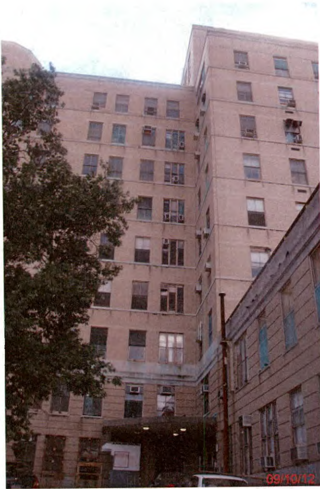
Southwest Rear View (3)
