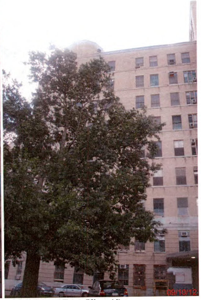
Southwest Rear View (4)
