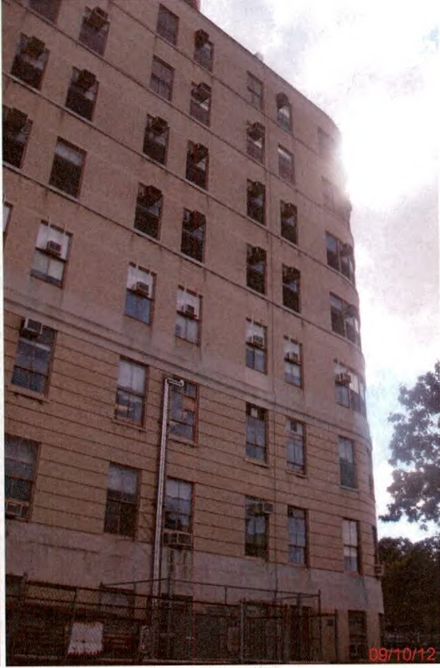
Southwest Rear View (8)
