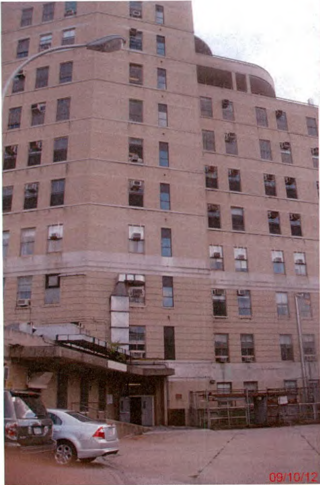
Southwest Rear View (7)
