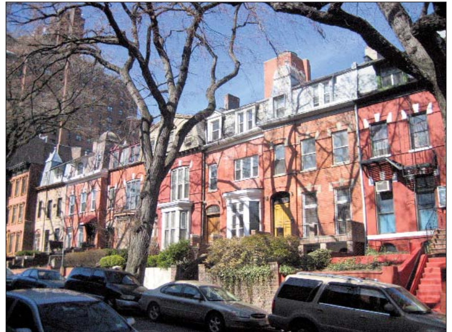
Above: View of northern blockfront of W. 145th Street between St. Nicholas and Amsterdam Avenues. (S/NR district and LPC Hamilton Heights/Sugar Hill HD & Extension)
