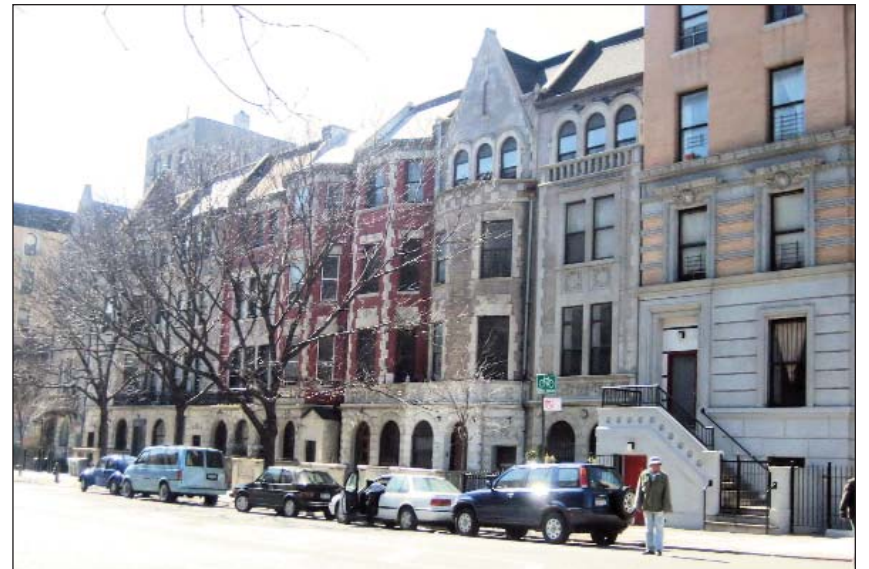
Below: View of western blockfront of St. Nicholas Avenue between W. 152nd and W. 153rd Streets. (S/NR district and LPC Hamilton Heights/Sugar Hill Northwest HD)
