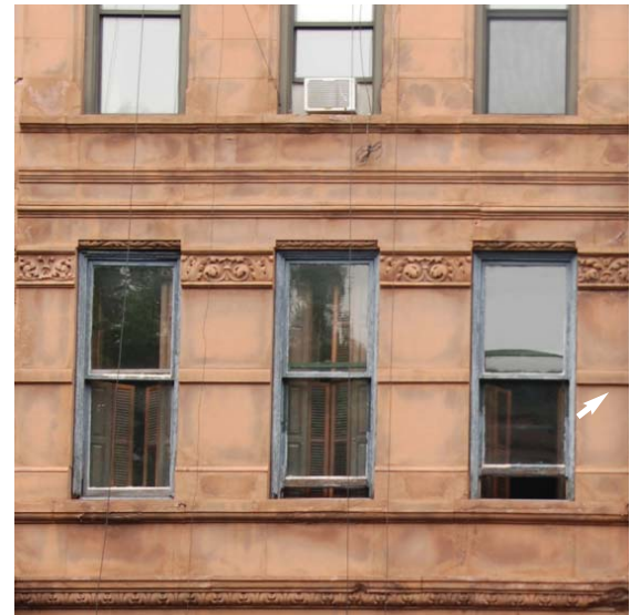
FLAT WITH CORNICE STRIPS
