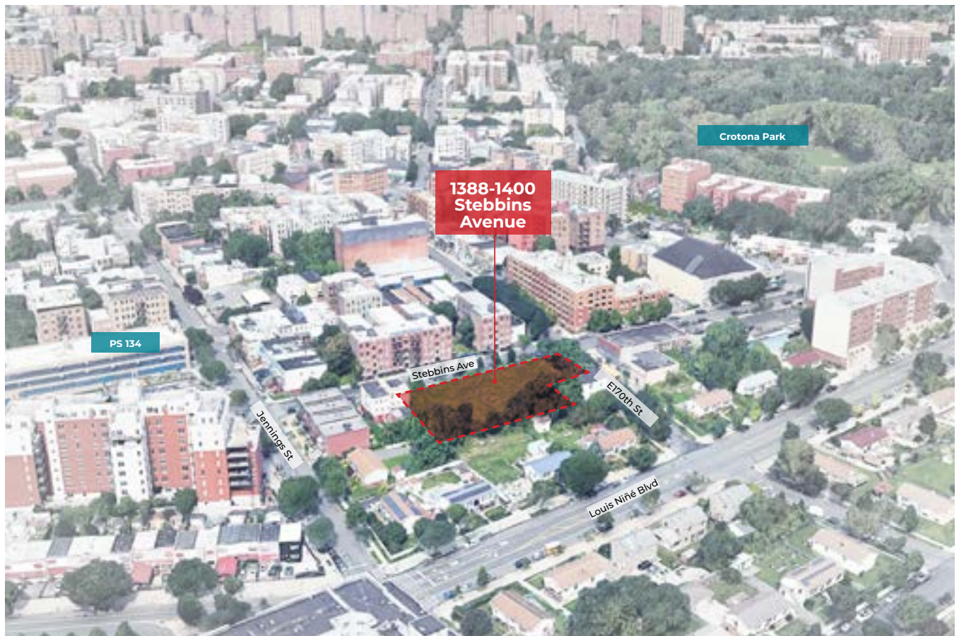
Site Aerial View
