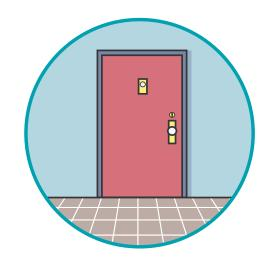
Apartment doors and hallway doors are required by law to swing closed and latch by themselves after being opened (self-closing) so that in the case of a fire no one needs to remember to close the door to trap the fire and smoke and stop it from spreading.
